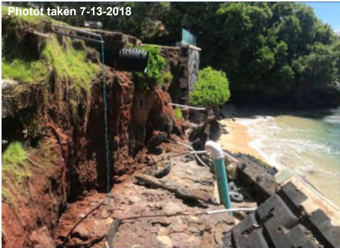
Figure 4-4. Hester shoreline facing south behind the portion of the retaining wall that collapsed
