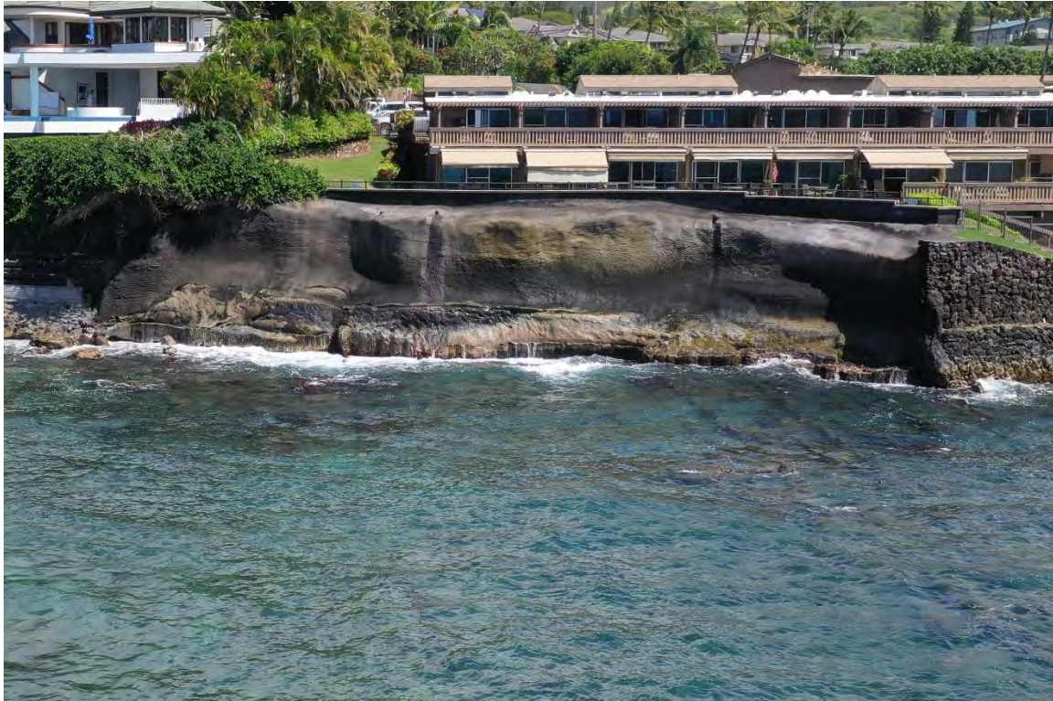
Figure 6-13. Example of shotcrete used over semi-lithified conglomerate on North side of project area Bay (Keonenui Bay, Maui)
