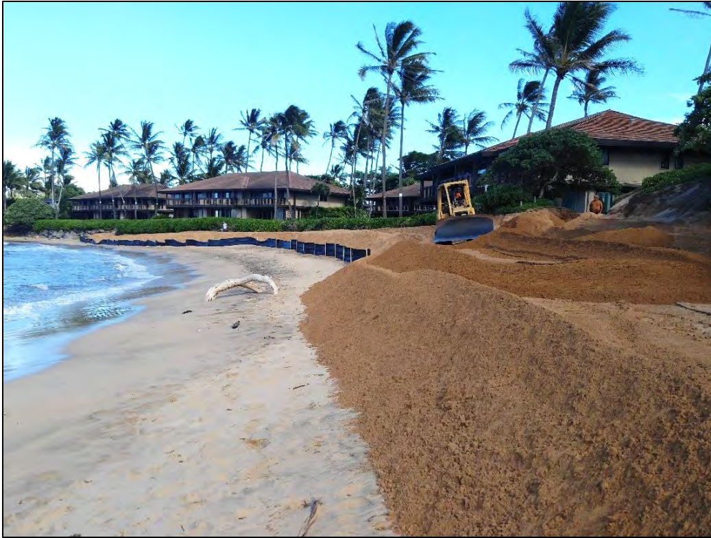
Figure 6-3. Small-scale beach nourishment at Sugar Cove (Paia, Maui)
