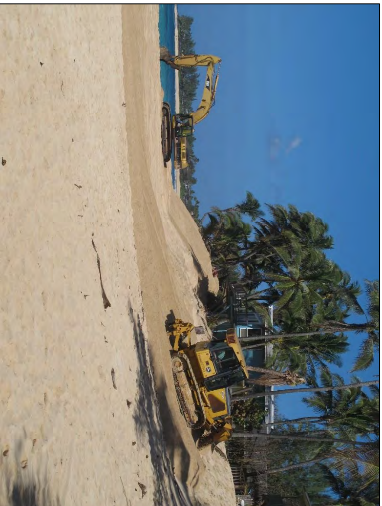
Figure 6-2. Sand pushing to build beach berm (Sunset Beach, Oahu)
