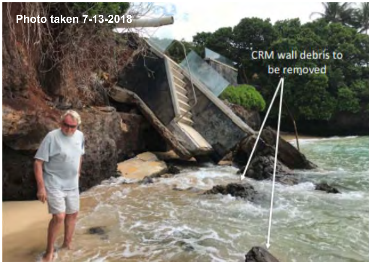
Figure 4-3. Hester shoreline after a portion of the retaining wall collapsed
