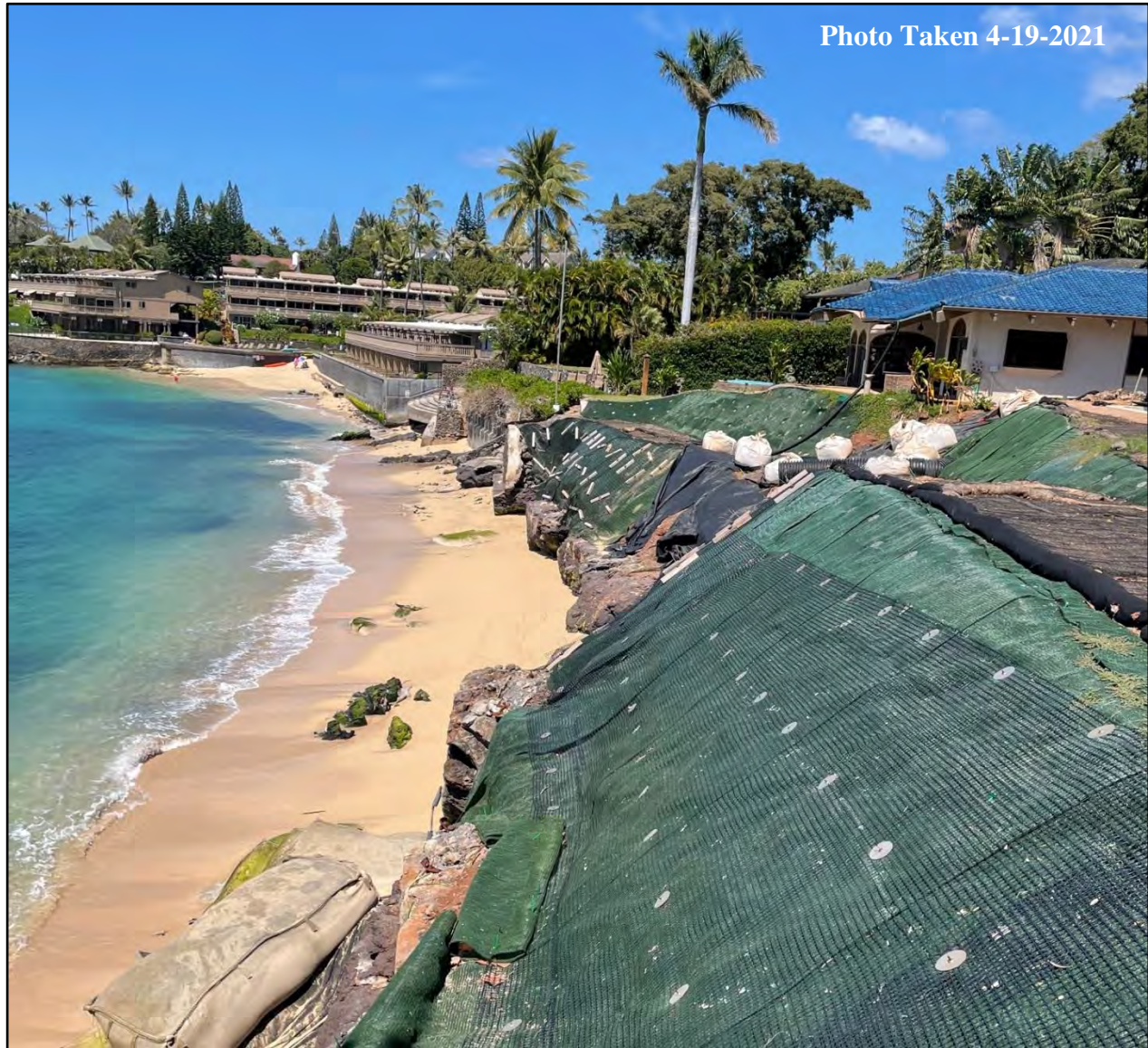
Figure 2-3. Slope stabilization in Keonenui Bay at the end of winter, facing north
