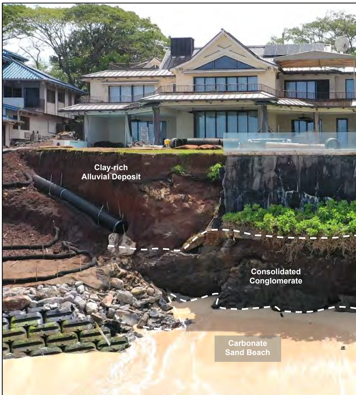
Figure 2-2. Cross-section of shoreline geology at the project site
