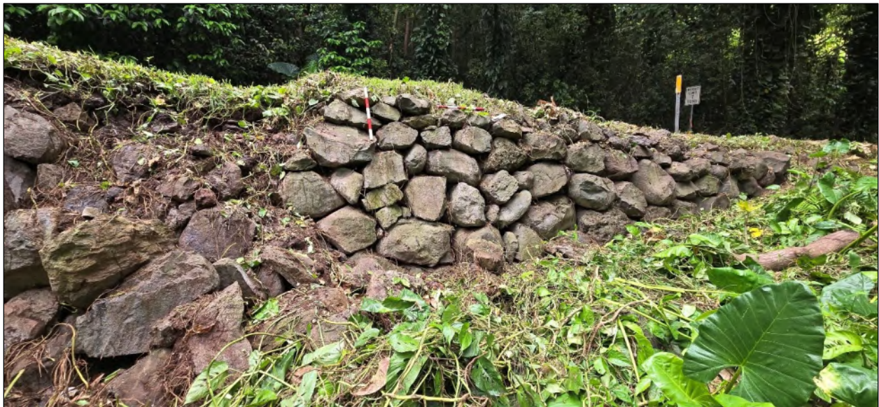
Figure 34. Another view of intact middle portion (center and right) of Feature 1, Hāna Belt Road south of South Wailua Bridge with collapsed south end (left); view northwest
