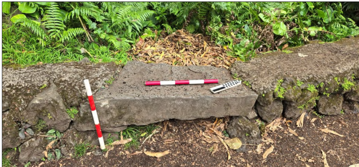
Figure 25. Detail of basalt slab repair near middle of Feature 1, South Wailua Bridge; view west-northwest
