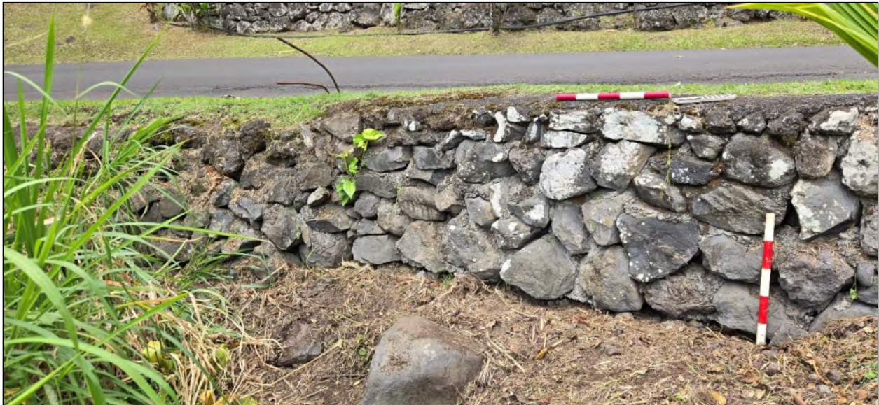
Figure 87. Detail of repaired portion of northern end of Feature 1, Hāna Highway at Waikakoi Bridge; original construction is to left of vertical rebar; facing west
