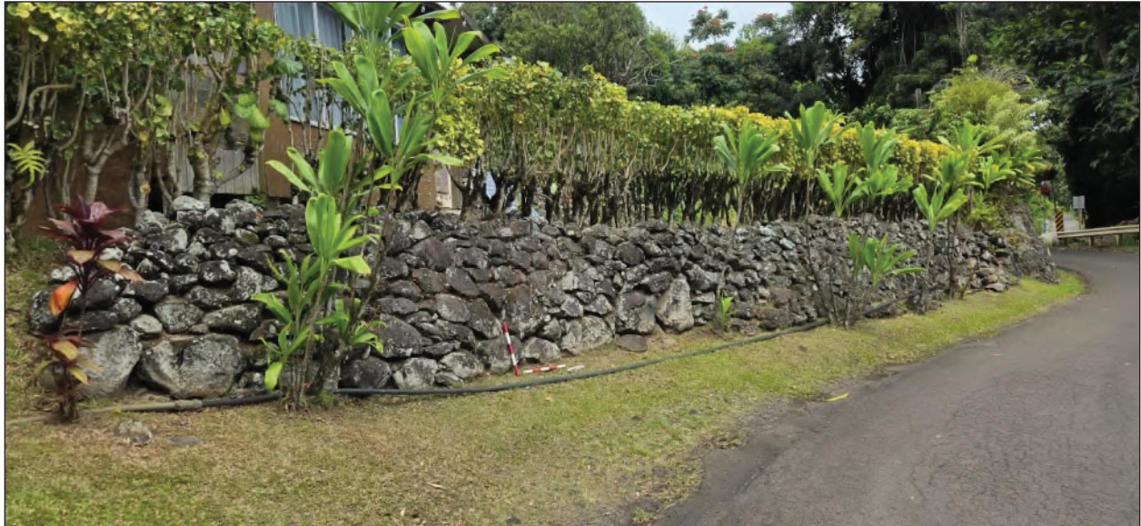
Figure 97. Overview of Site, dry-stacked rock retaining wall along mauka shoulder south of Waikakoi Bridge (see text above for discussion); facing northwest
