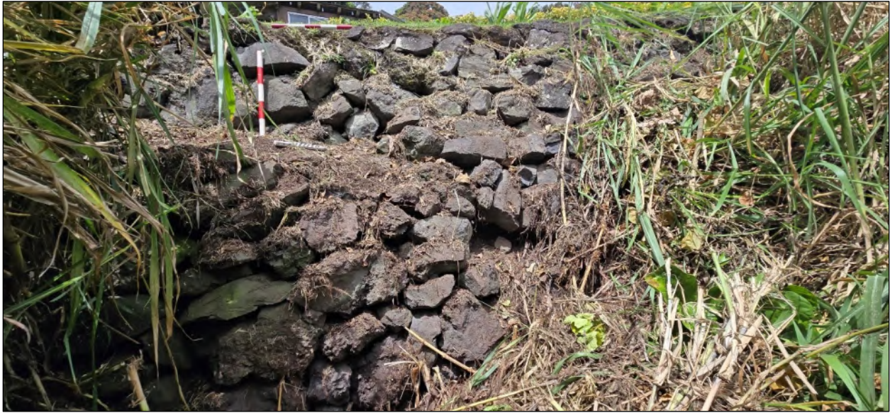
Figure 88. Detail of two-level retaining wall construction at Feature 1, Hāna Highway at Waikakoi Bridge; view west
