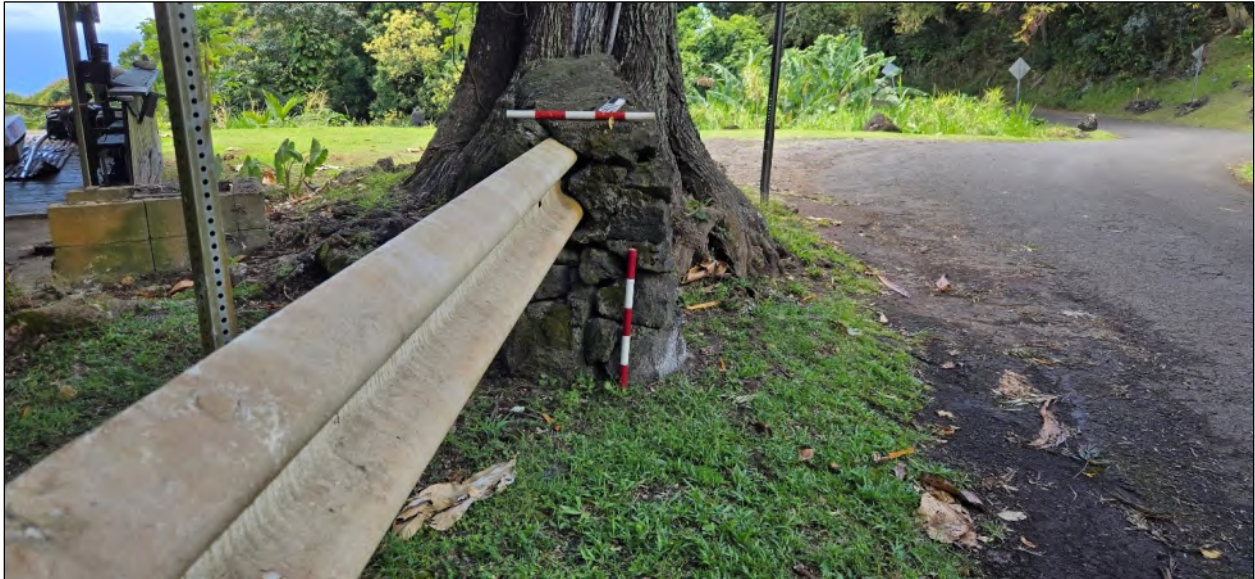
Figure 82. Overview of Feature 6, Waikakoi Bridge built around and as an anchor to guardrail; view south
