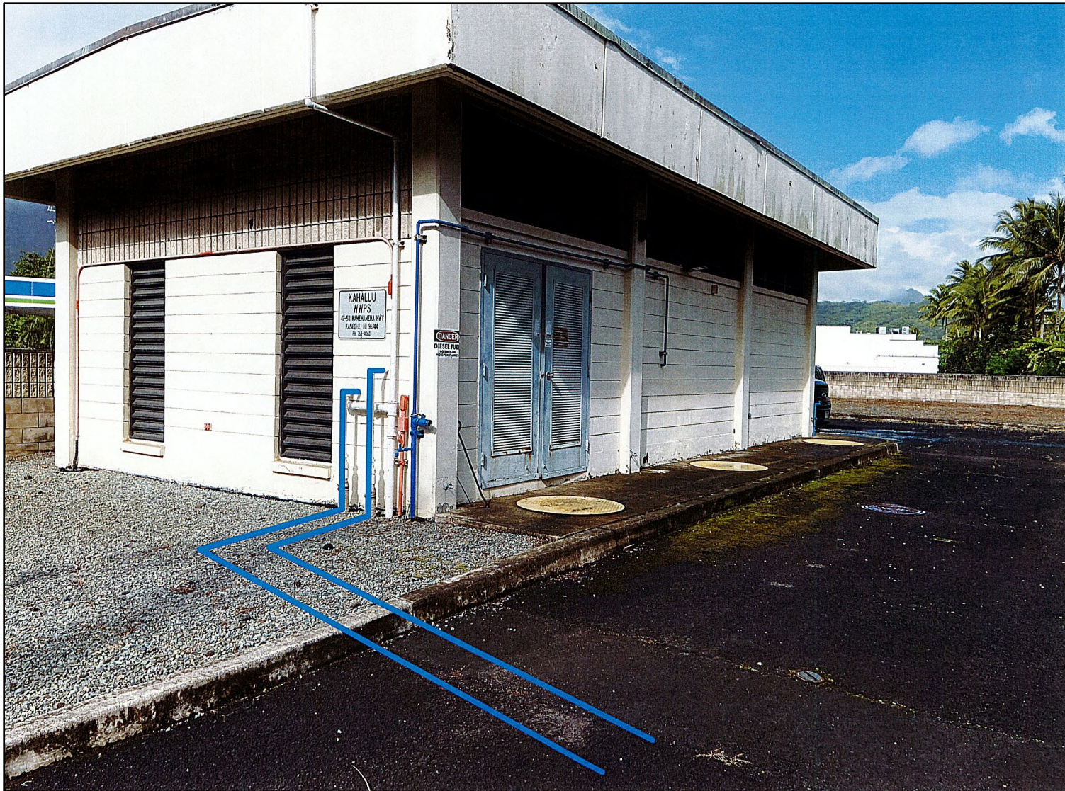
Figure 6. Indicated route of underground fuel piping approaching the Kahaluu WWPS building (Okahara and Associates, Inc.; courtesy of client)
