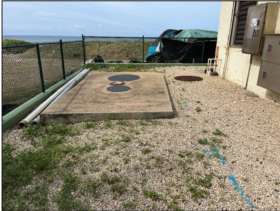
Figure 41. Photo K: View of the proposed location of new 2,000-gallon Convault aboveground fuel storage tank (at location of existing UST at concrete slab) in south corner of Lualualei WWPS, view to southwest
