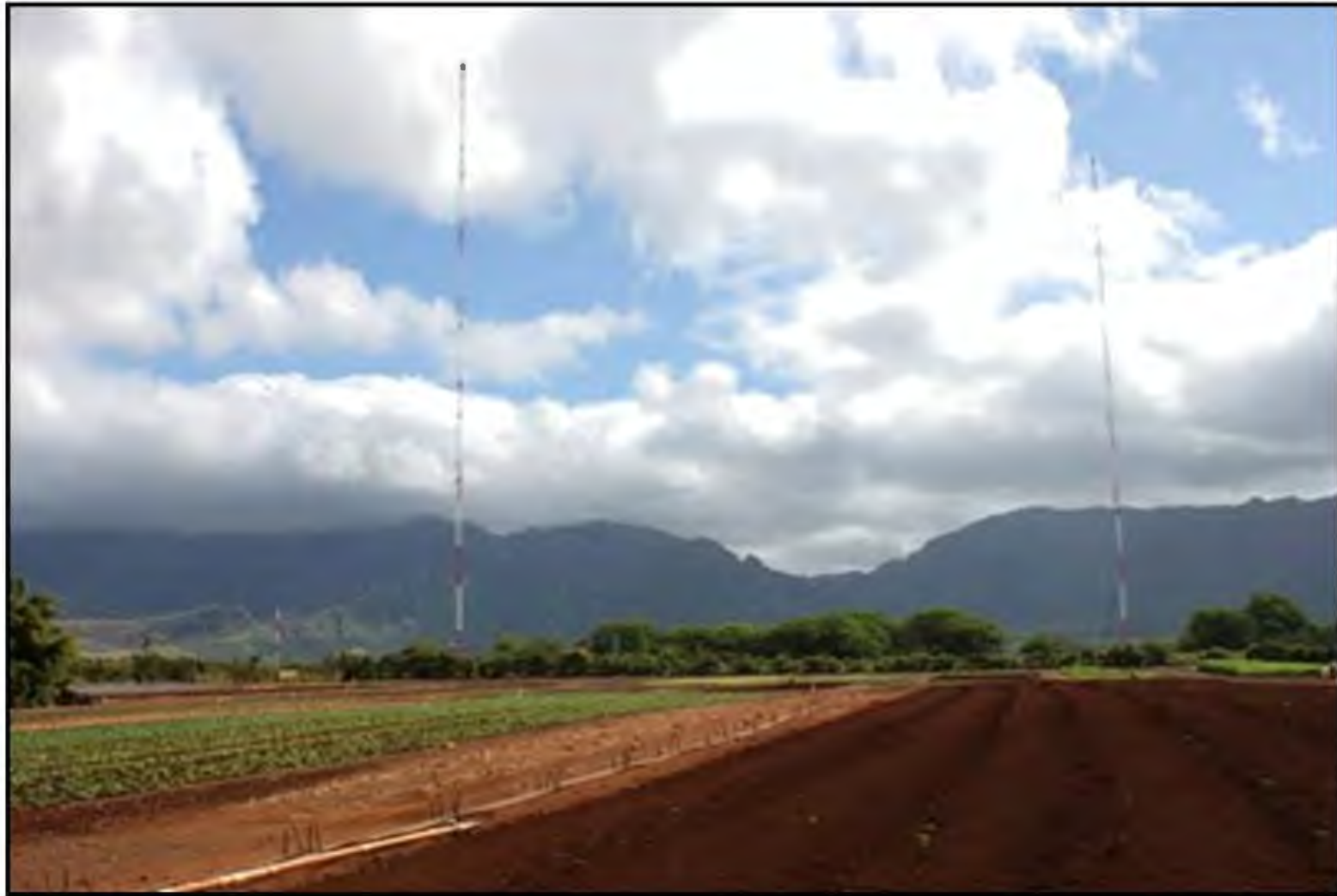
Figure 27. Photo of the two antennas used for the Navy's communication systems at Lualualei; the two antennas stand at 1,503 ft, the highest structures in the State of Hawai'i (CSH 2012)
