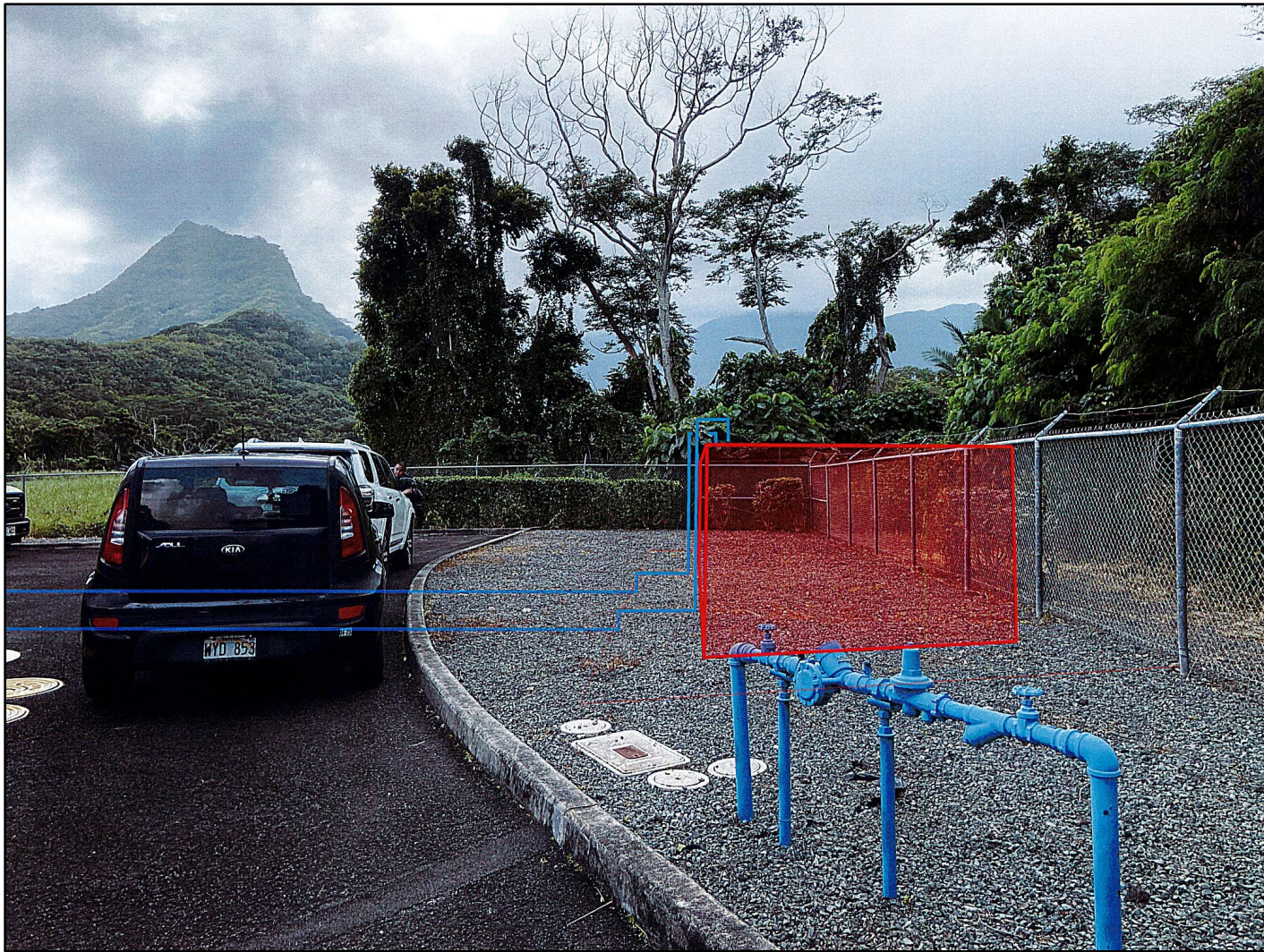
Figure 5. Photograph showing the location of the new 1,000-gallon AST on the central west side of the Maunawili Park Wastewater Pump Station facility and adjacent new underground fuel piping, view to south (Okahara and Associates, Inc.; courtesy of client)
