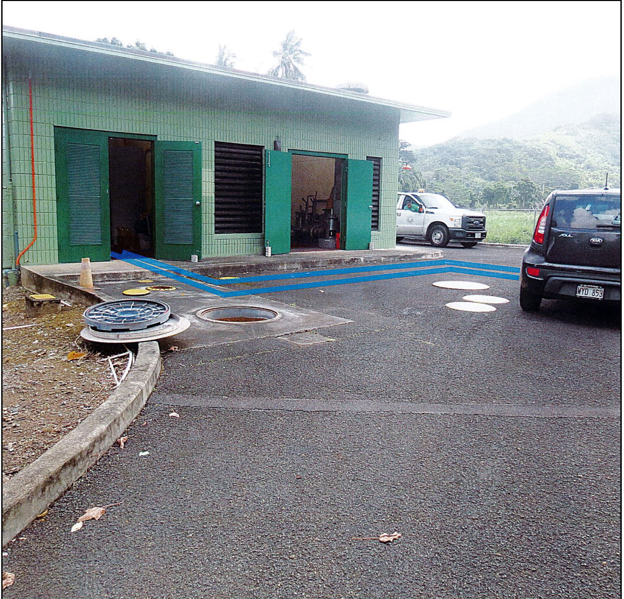
Figure 6. Photograph showing the location of new underground fuel piping as it enters existing pump station building, view to south (Okahara and Associates, Inc.; courtesy of client)
