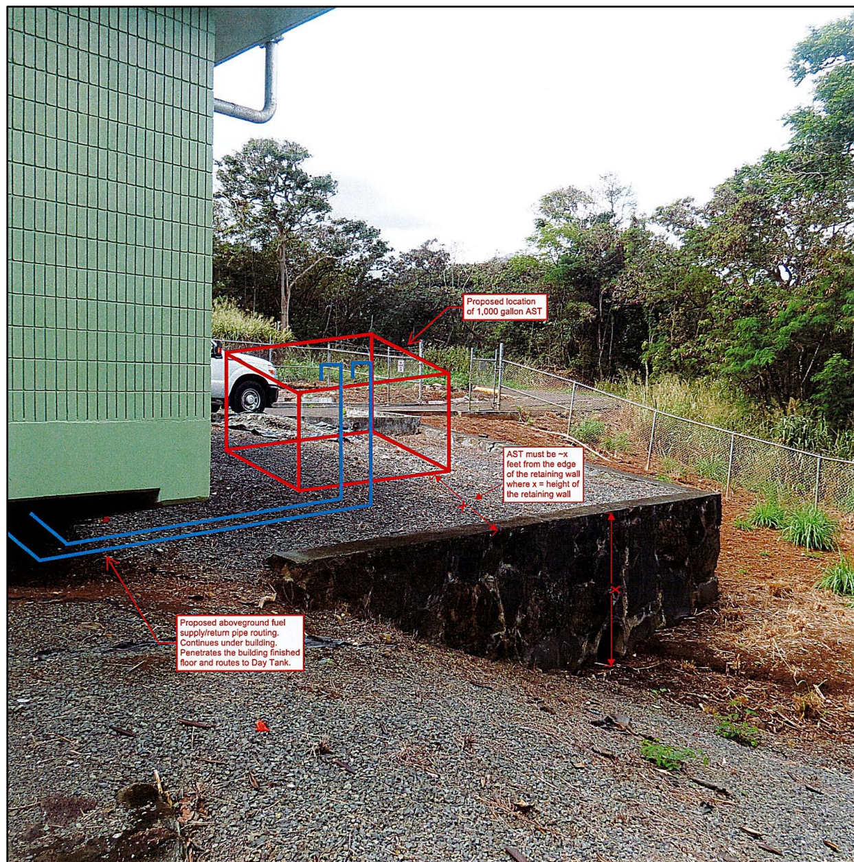
Figure 5. Photo showing proposed location of the proposed 1,000-gallon AST and proposed fuel supply and return pipe routing at the Kukanono WWPS (Okahara and Associates, Inc.; courtesy of client)
