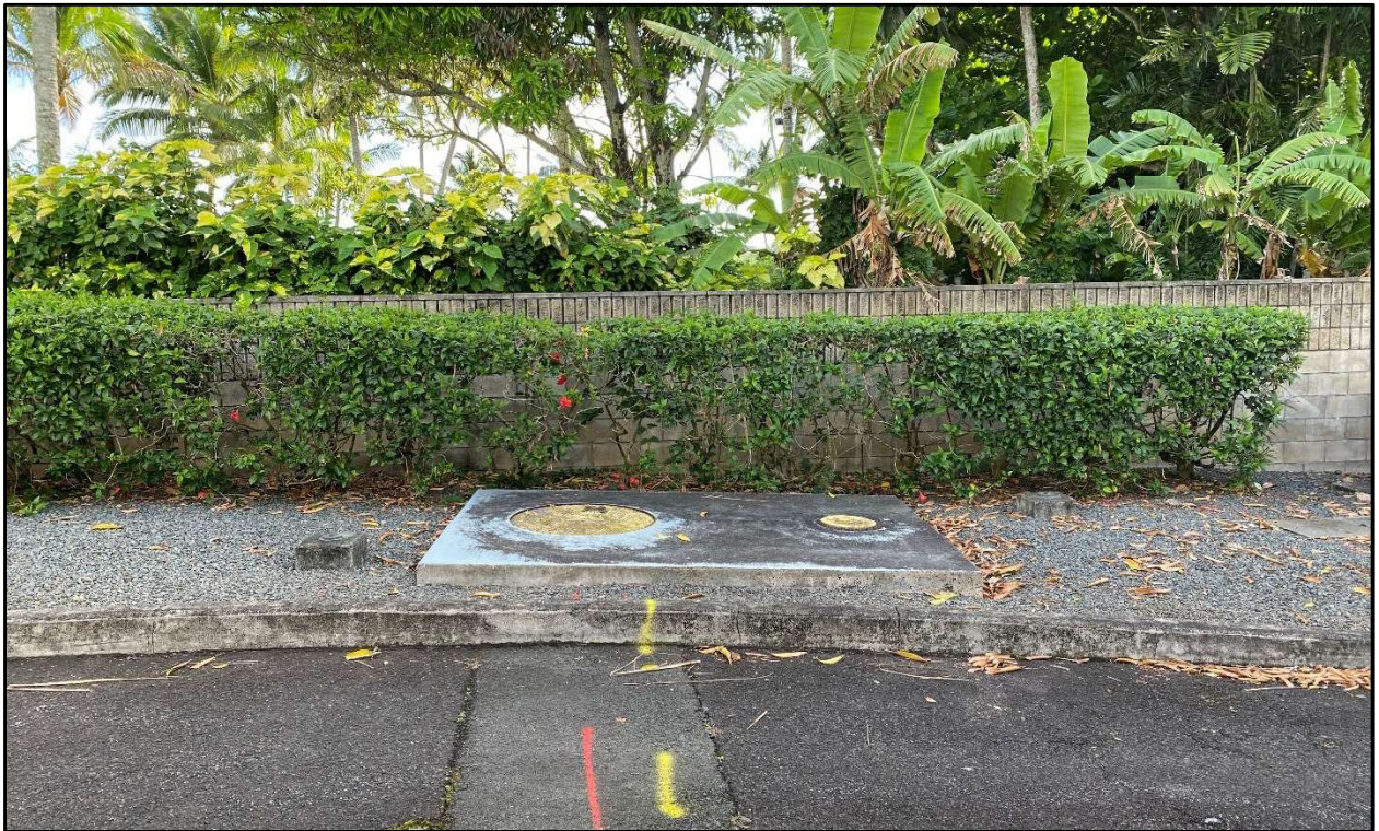
Figure 37. Photo H: View of existing underground storage tank, view to east
