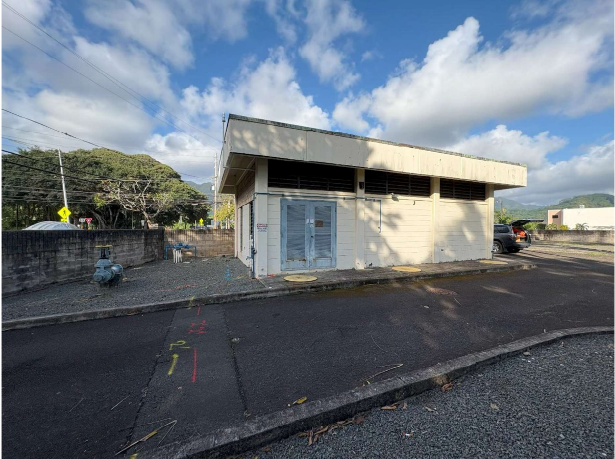
View of the WWPS (from the driveway)
