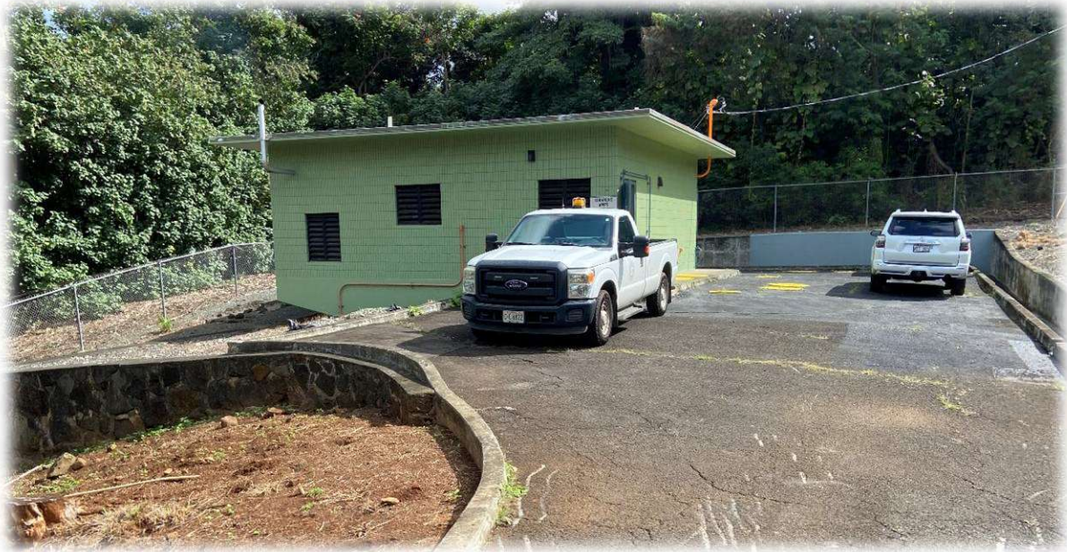
View of the WWPS (from the driveway)
