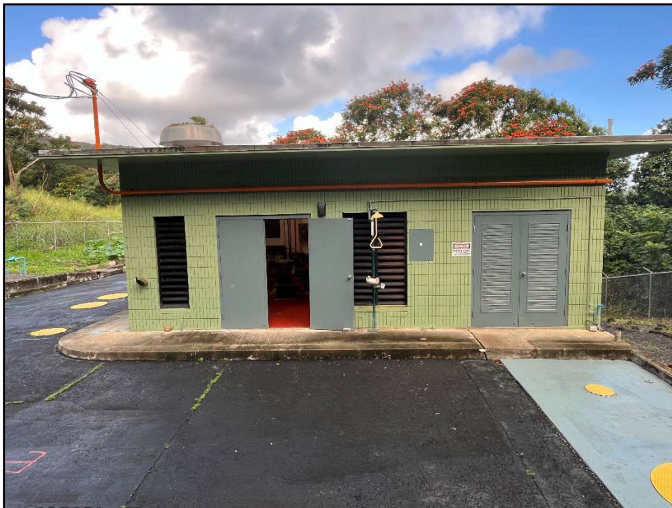
Figure 37. Photo F: View of the front (entrance on southeast side) to the Kukanono WWPS Building, view to northwest
