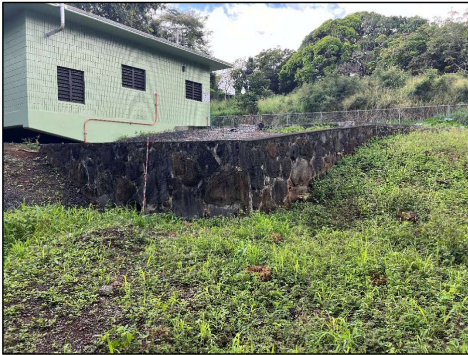
Figure 51. Photo T: View of the corner of the retaining wall at the Kukanono WWPS facility under evaluation for repair/replacement, view to south
