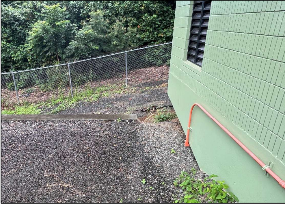
Figure 46. Photo O: View of proposed fuel supply and return pipe routing at northwest corner of the Kukanono WWPS Building, view to northeast
