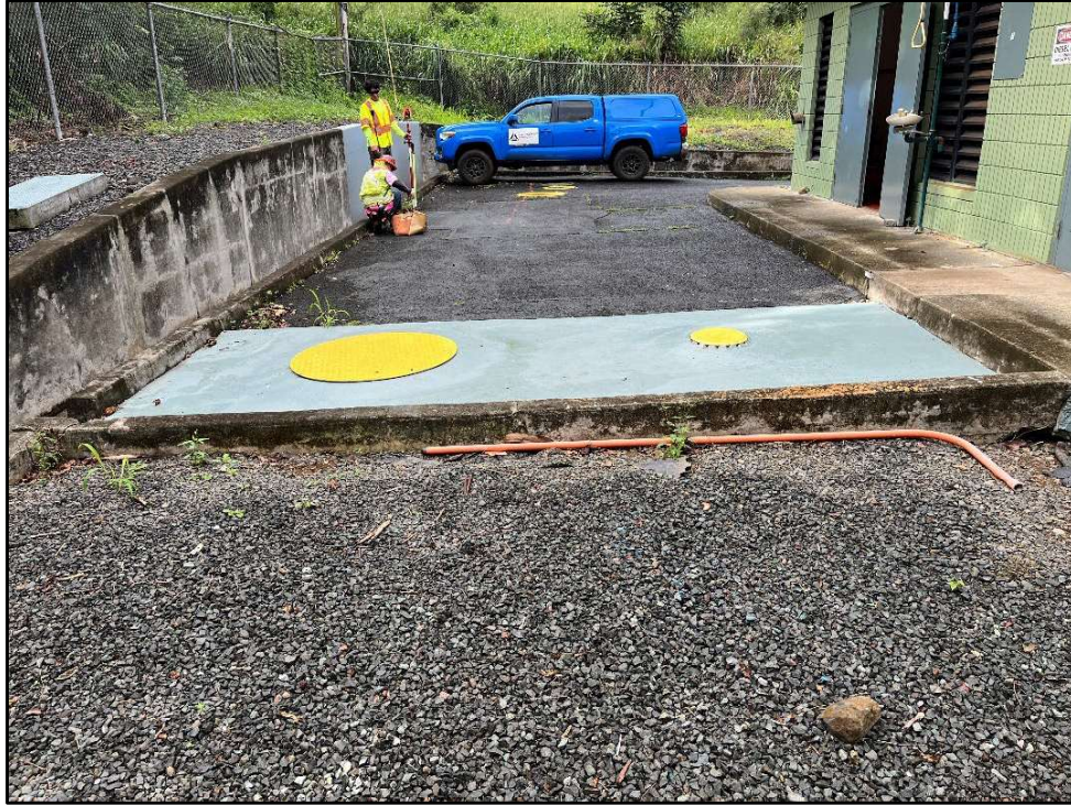
Figure 42. Photo K: View of the location of the existing 1,000-gallon UST (under concrete slab) at the northeast corner of the Kukanono WWPS Building, view to southwest
