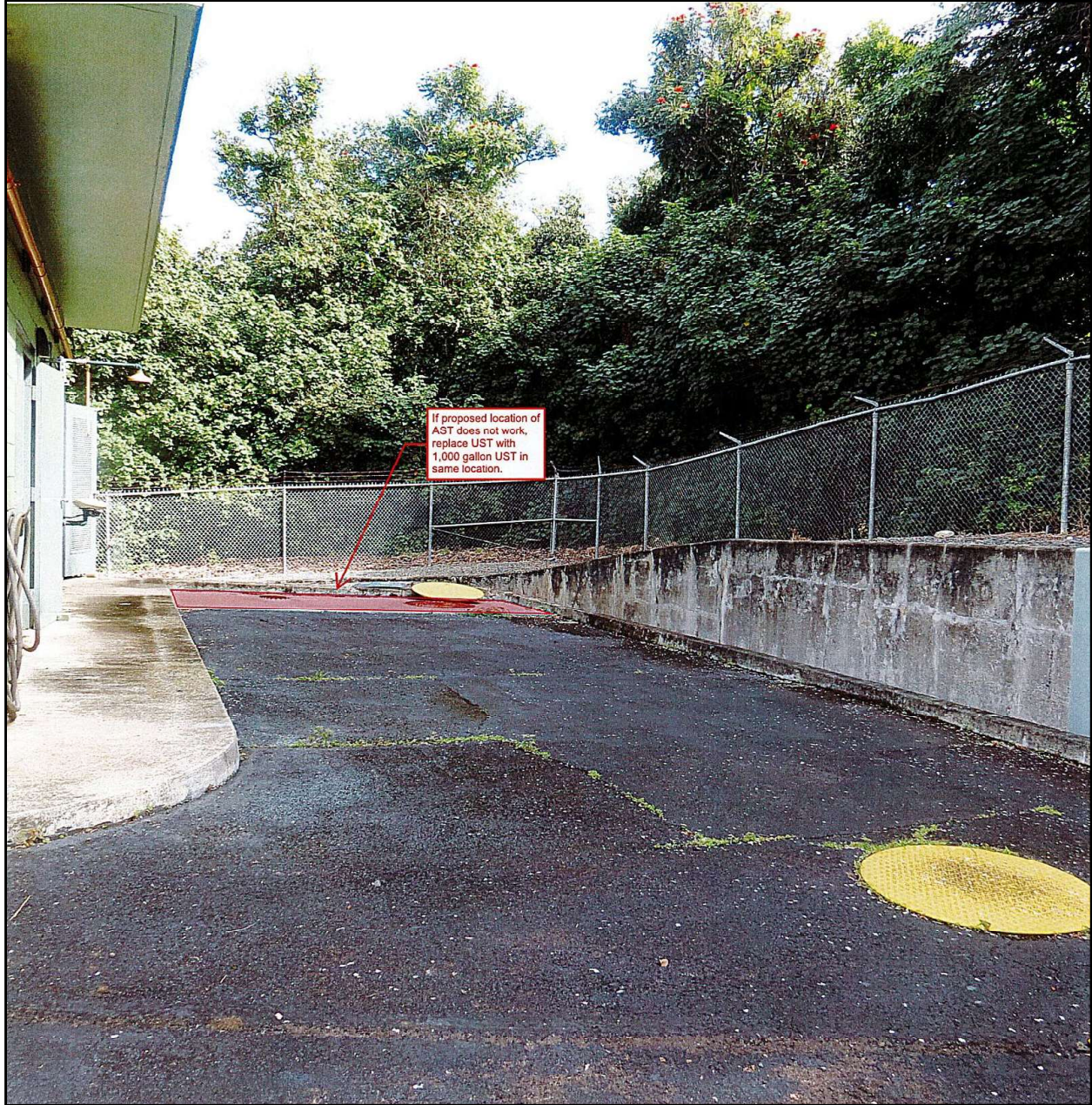
Figure 7. Photo showing proposed location if AST does not work and the alternative is to replace the existing UST with a new 1,000-gallon UST in the same location at the Kukanono WWPS (Okahara and Associates, Inc.; courtesy of client)
