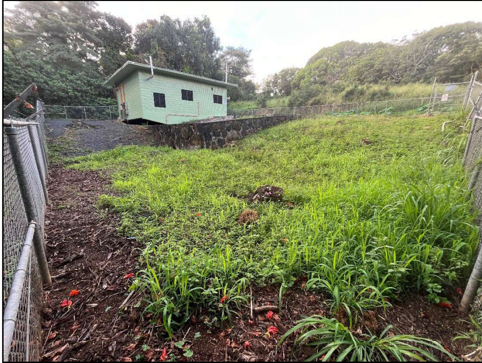
Figure 36. Photo E: View of the Kukanono WWPS facility from the northwest corner, view to southeast
