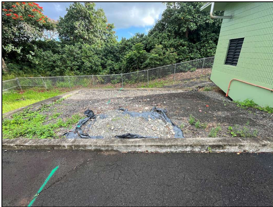
Figure 43. Photo L: View of the proposed location of a new 1,000-gallon UST (northwest of the Kukanono WWPS Building), view to northeast
