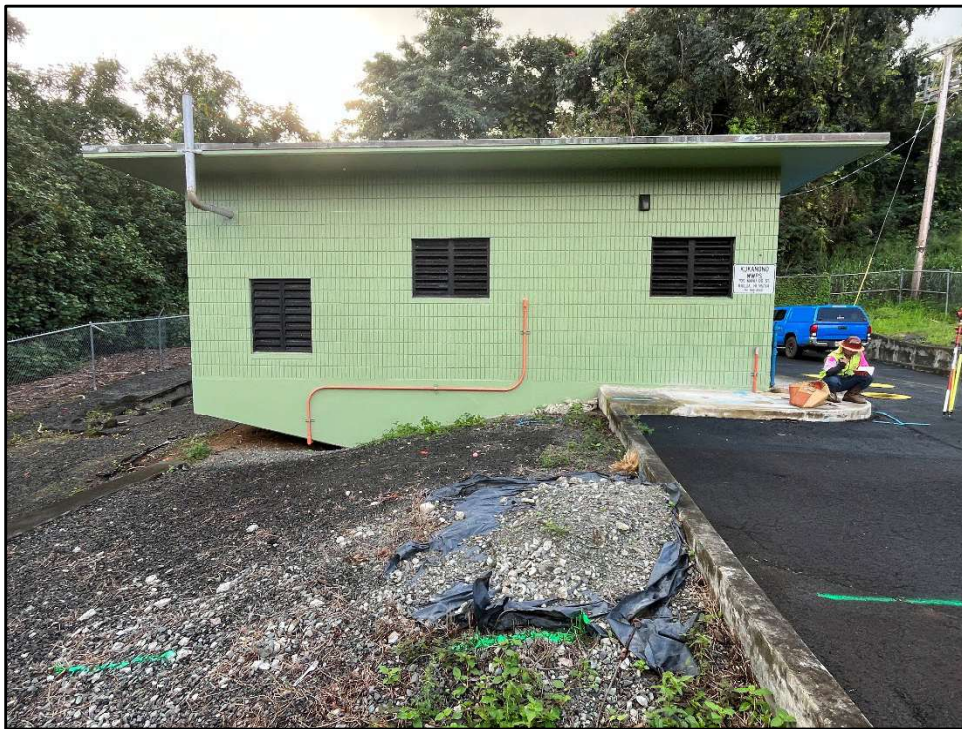
Figure 39. Photo H: View of the northwest side to the Kukanono WWPS Building, view to southeast
