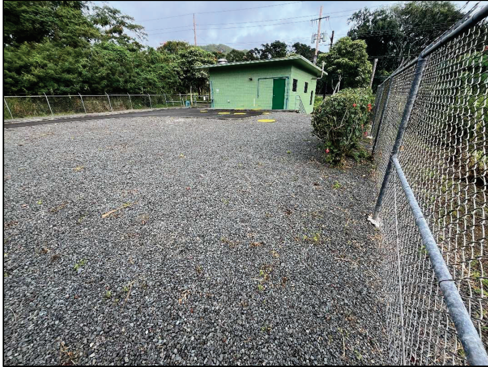
Figure 34. Photo C: View of the Maunawili Park WWPS from the southeast corner of the enclosure, view to northwest
