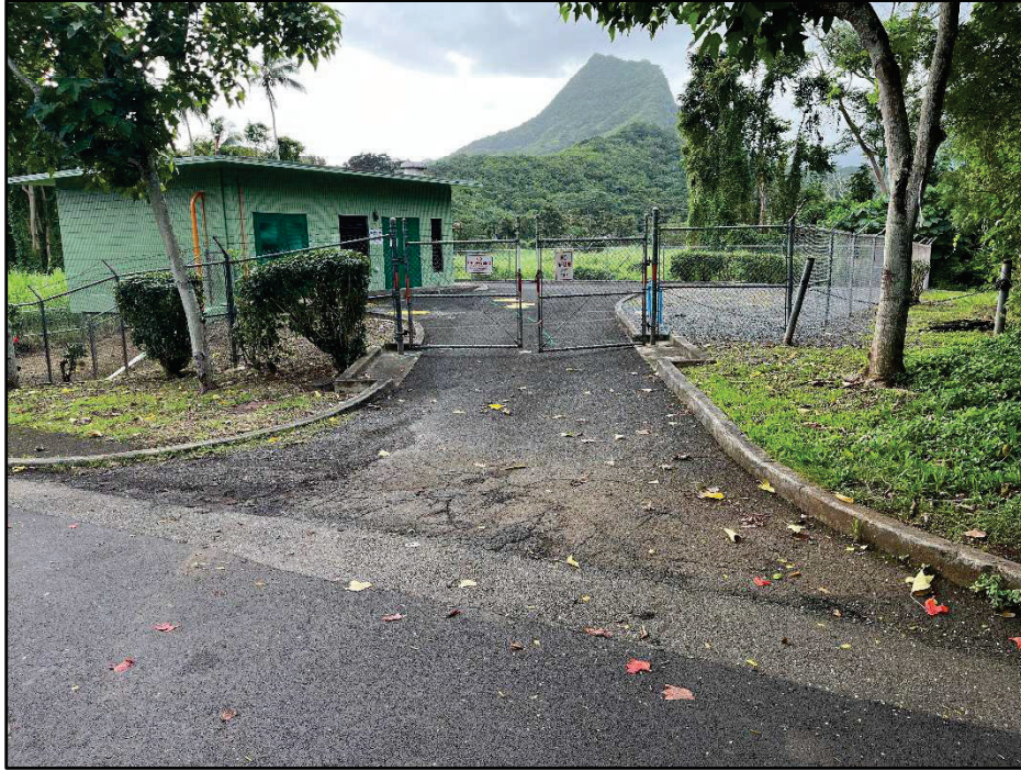
Figure 32. Photo A: Entry driveway to the Maunawili Park WWPS; the proposed AST is to be located in the gravel area on the west side of the facility (at right), view to southeast
