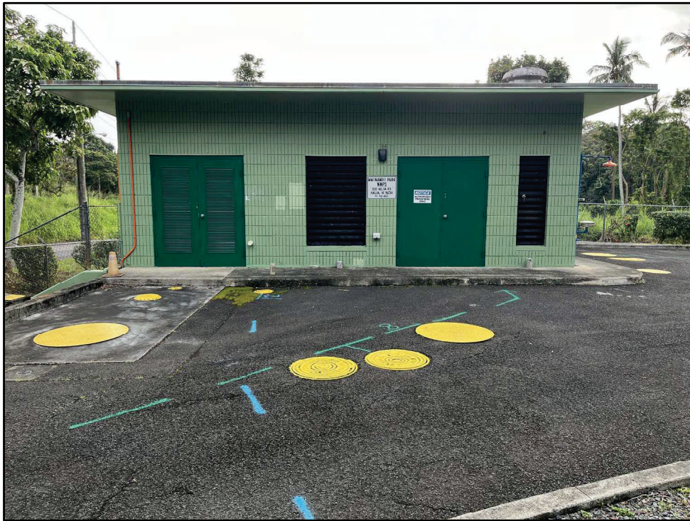
Figure 37. Photo F: View of the front (west side) of the existing Pump Station building, view to east
