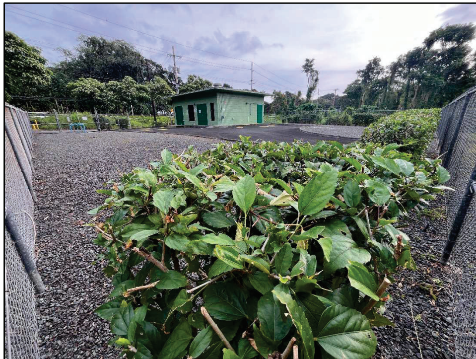
Figure 35. Photo D: View of the Maunawili Park WWPS from the southwest corner of the enclosure, view to northeast
