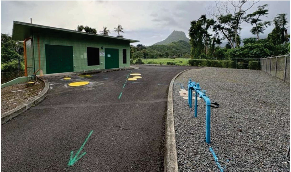
Figure 12 Maunawili Park WWPS as seen from Auloa Road
