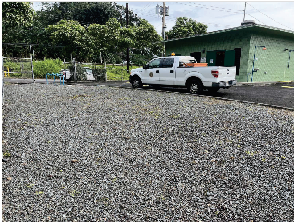
Figure 43. Photo L: View of the area of the proposed new underground fuel piping from the new 1,000-gallon AST (at left) to the existing Pump Station, view to northwest
