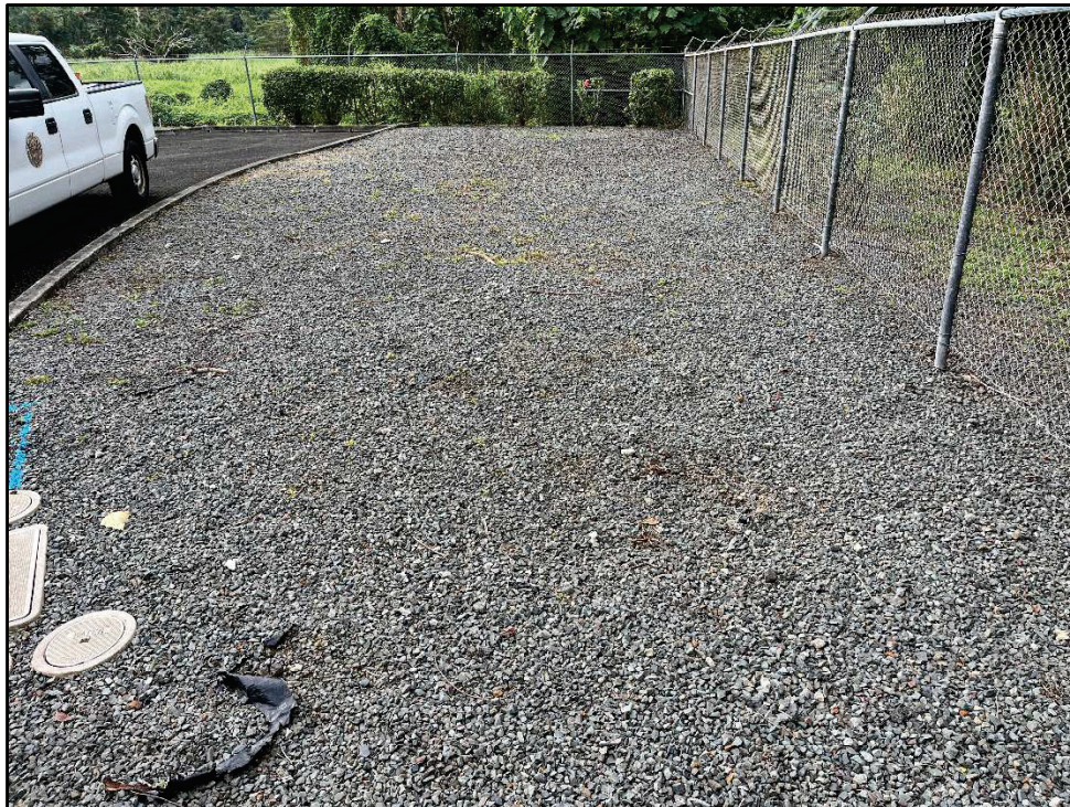
Figure 41. Photo J: Location of proposed new 1,000-gallon AST in the west side of Maunawili Park WWPS enclosure, view to southeast
