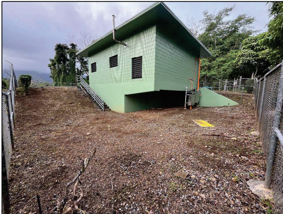
Figure 33. Photo B: View of the Maunawili Park WWPS from the northeast corner of the enclosure, view to southwest
