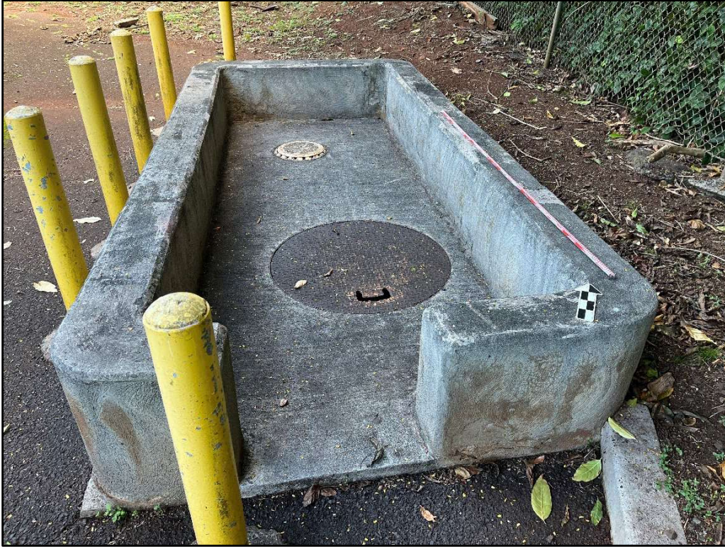
Figure 34. Photo I: View of existing 1,000-gallon diesel UST, view to northwest
