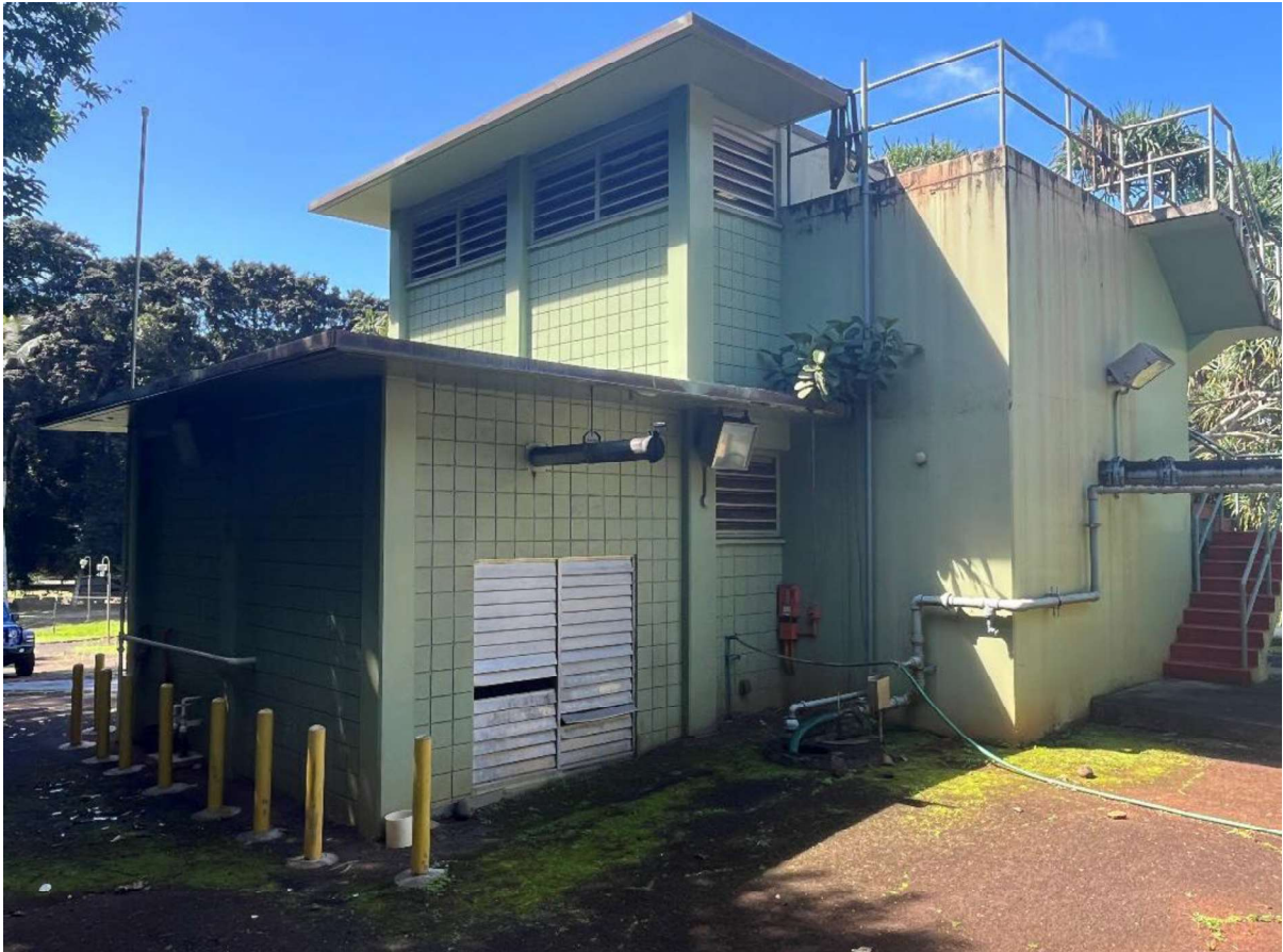
View of WWPS and location of the proposed AST to the right of the facility (in the cleared area).
