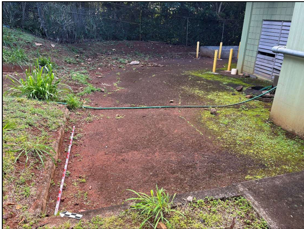
Figure 37. Photo L: View of area for the proposed AST installation, view to northeast
