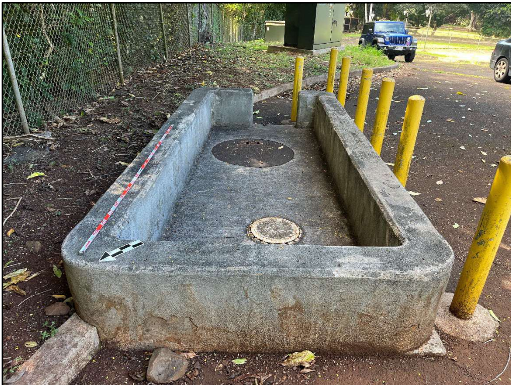
Figure 35. Photo J: View of existing 1,000-gallon diesel UST, view to southeast
