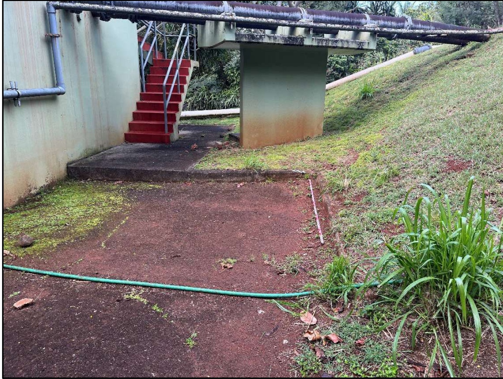
Figure 36. Photo K: View of area for the proposed AST installation, view to southwest
