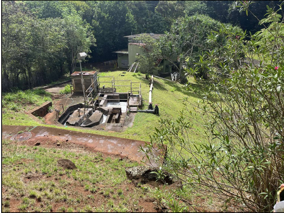
Figure 28. Photo C: View from the northwest corner of the Pacific Palisades WWPS facility, view to southeast
