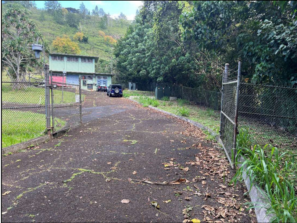
Figure 26. Photo A: View of entry gate into the Pacific Palisades WWPS facility, view to northwest
