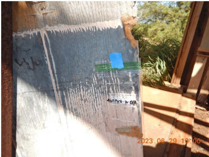
Photo 19 - 4011PKA-W-01A (Close-up) [BB\DSCN9838.JPG]
