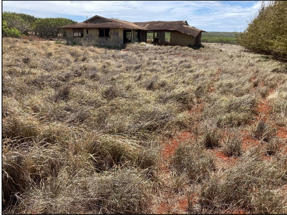
Figure 34. Photo G: General view of the 4.7-acre TMK: [2] 5-2-026:014 parcel from the northwest corner, view to southeast
