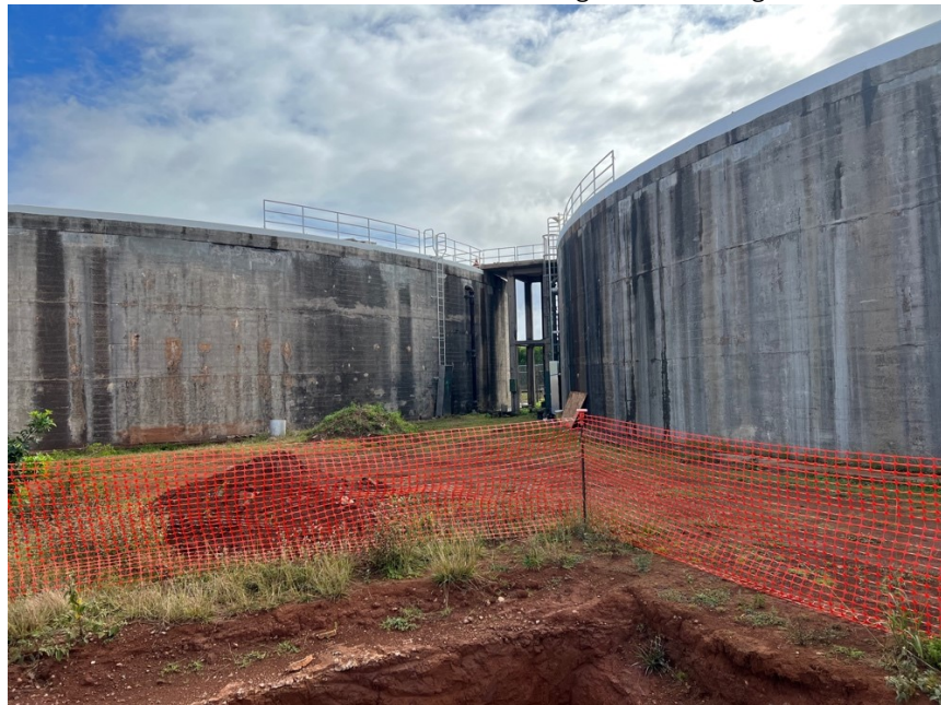
Picture 4. Site #4 water tank upgrades and valve replacements.
