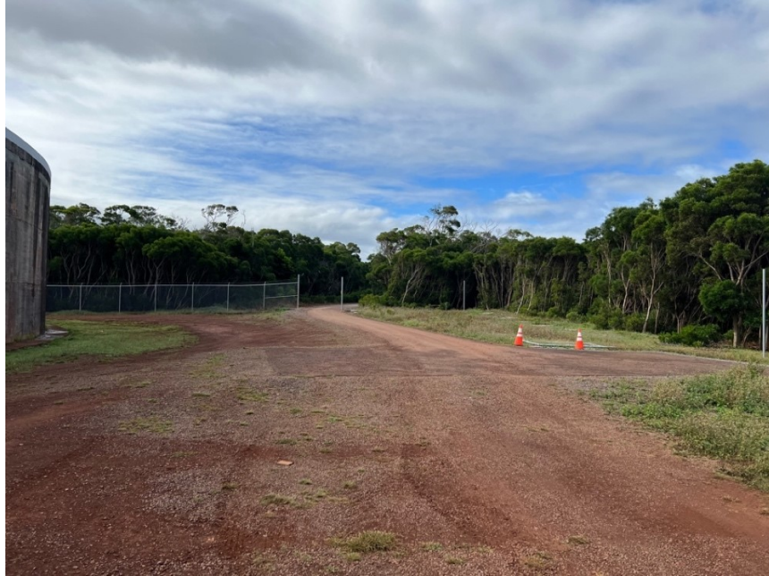
Picture 5. New 8-foot fenceline installation at Site #4
