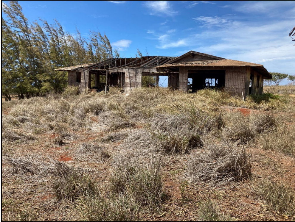
Figure 38. Photo K: General view of the abandoned house in the 4.7-acre TMK: [2] 5-2-026:014 parcel, view to northwest
