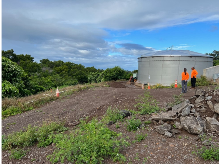
Picture 3. Site #1 water tanks and retaining wall to the right of tank.
