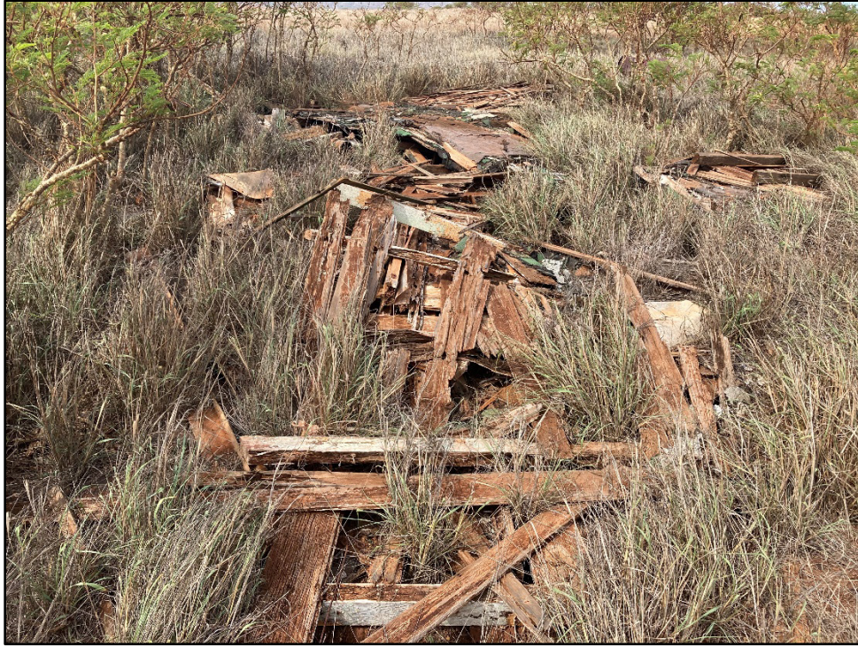
Figure 31. Photo E: View of collapsed structure in the 31.7-acre TMK: [2] 5-2-005:031 parcel, view to southwest
