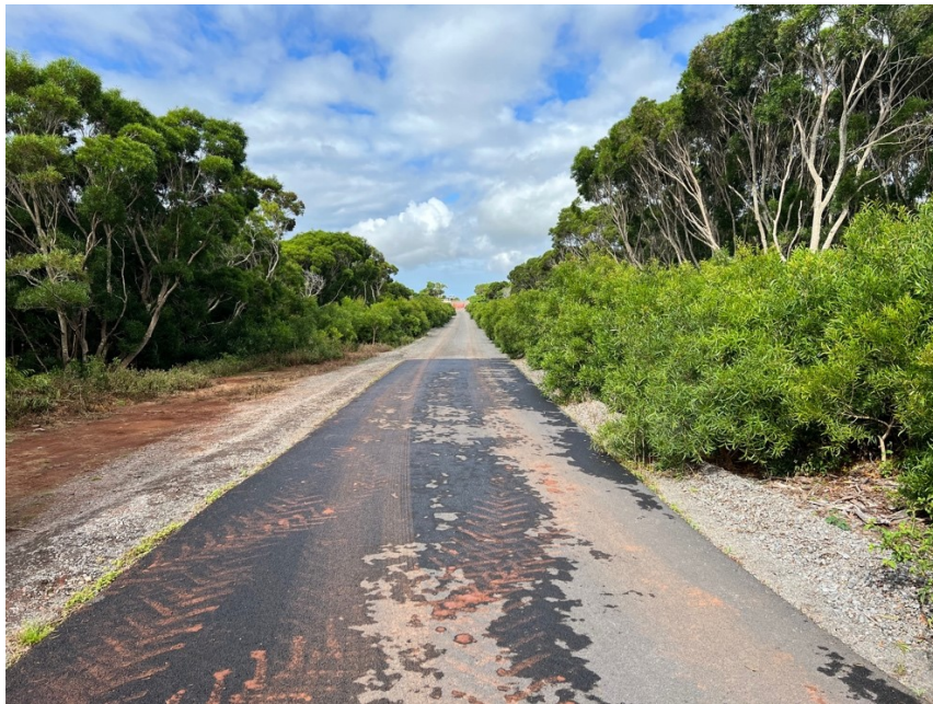
Picture 6. New access road at Site #4
