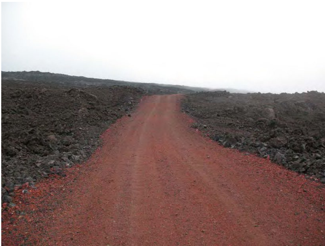
Figure 7. Typical view of existing graded and cindered access road.
