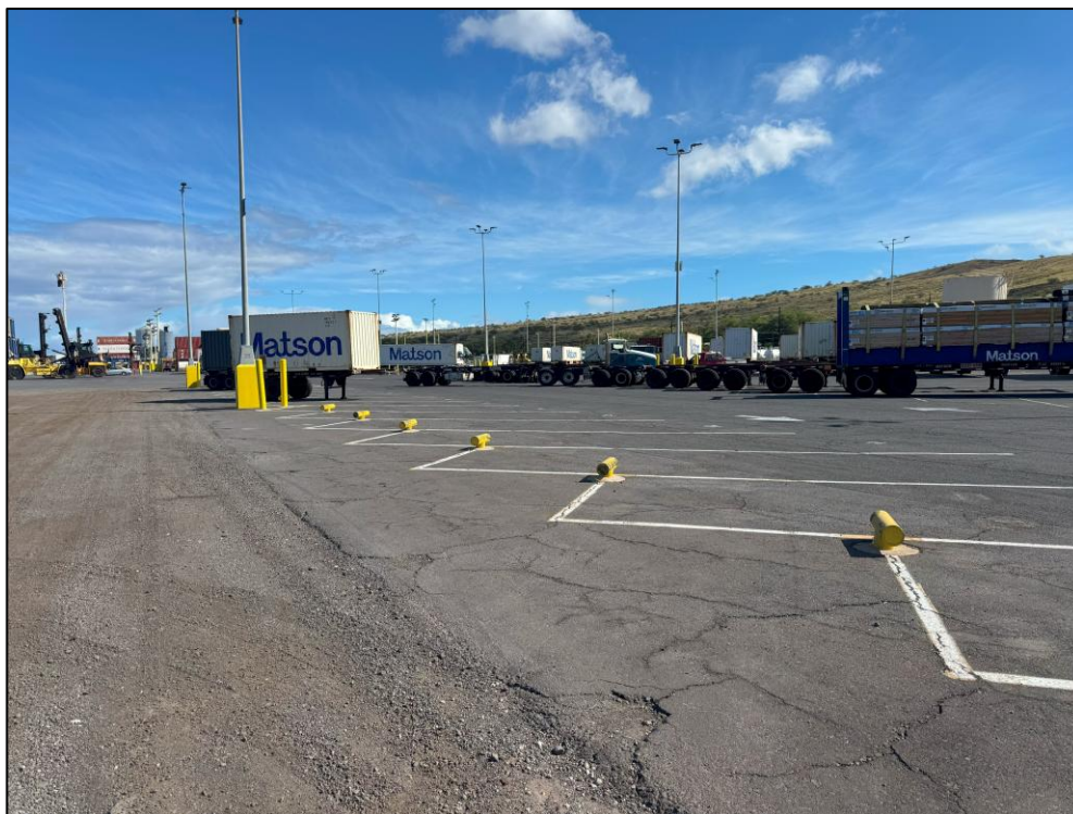
Figure 2. A trailer parking area at Kawaihae Harbor.
