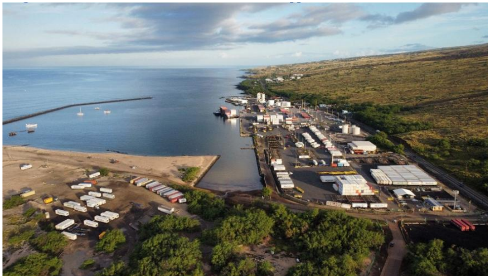
Figure 3-6. Aerial View of the Project Site Looking North
