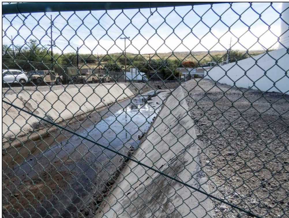
Figure 4. Concrete-lined open culvert crossing the Project APE.
