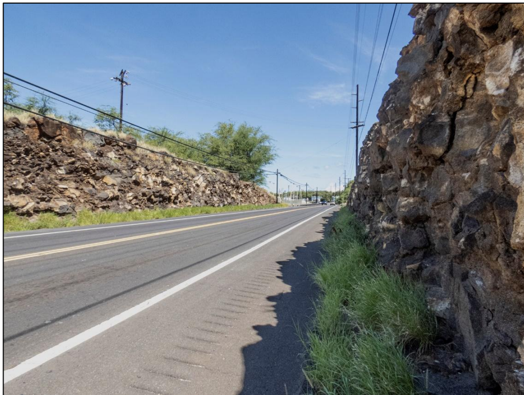
Figure 6. Kawaihae Road at cut showing verge vegetation.
