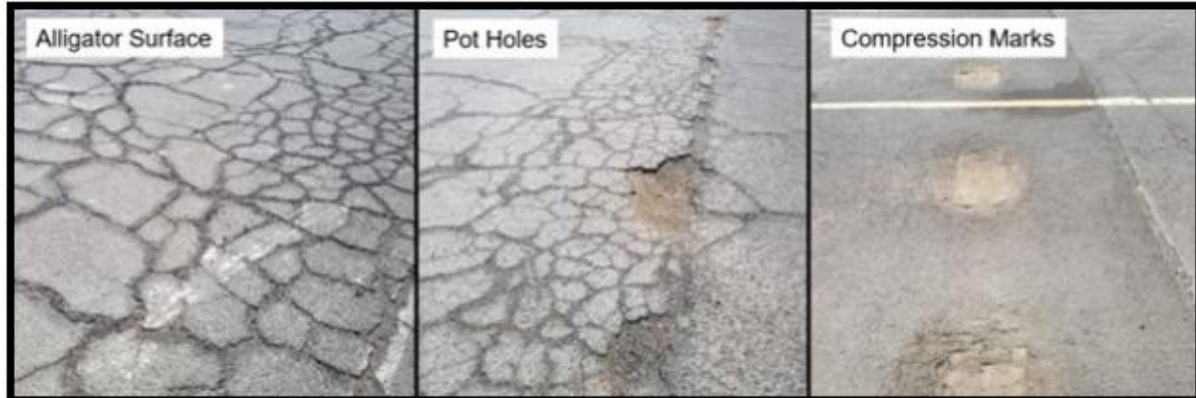
Figure 1-9. Asphalt Surface Conditions at Kawaihae Harbor
