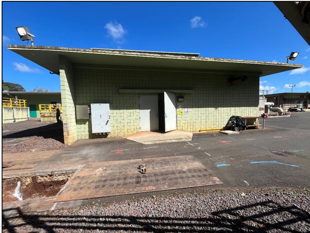
Figure 31. Photo F: Front of generator building, (project area at left), view to northwest
