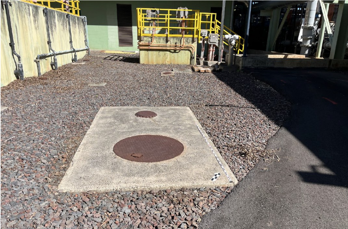
Existing UST (at cement slab); proposed AST area in background
