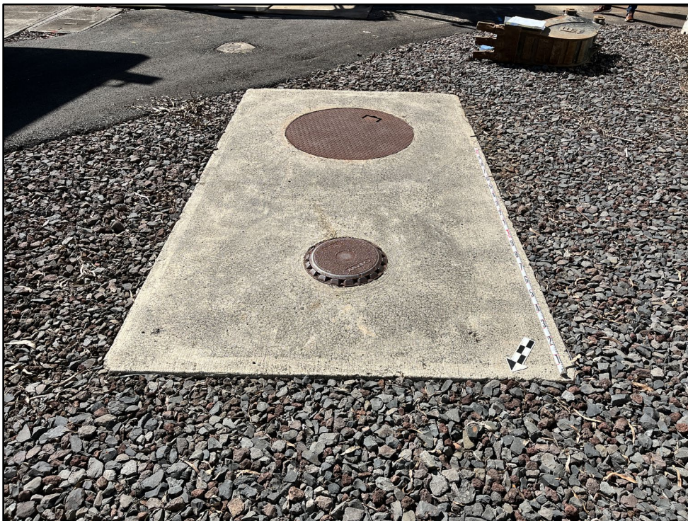
Figure 27. Photo B: View of the immediate area of the 6,000-gallon diesel UST (at cement slab) to be removed, view to southeast
