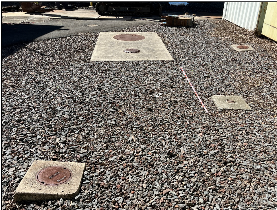
Figure 29. Photo D: Immediate area proposed for new 6,000-gallon diesel AST in foreground (existing UST in background), view to southeast
