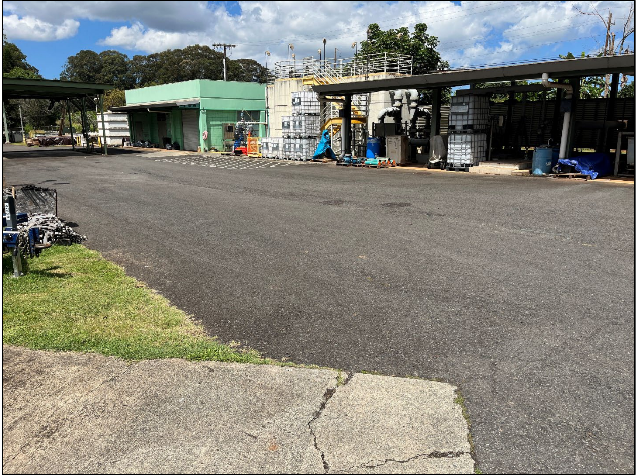
Figure 40. Photo O: General view of the central portion of the Wahiawa WWTP, view to northwest
