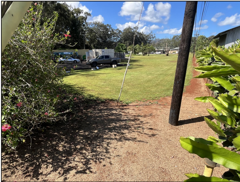
Figure 33. Photo H: General view of the Wahiawa WWTP from the north corner (near the entrance gate), view to southwest
