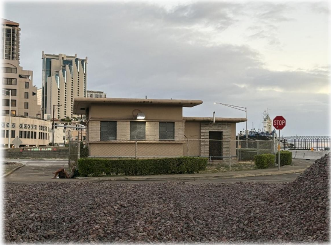
Figure 3 View of the Awa Street WWPS Facing Downtown
