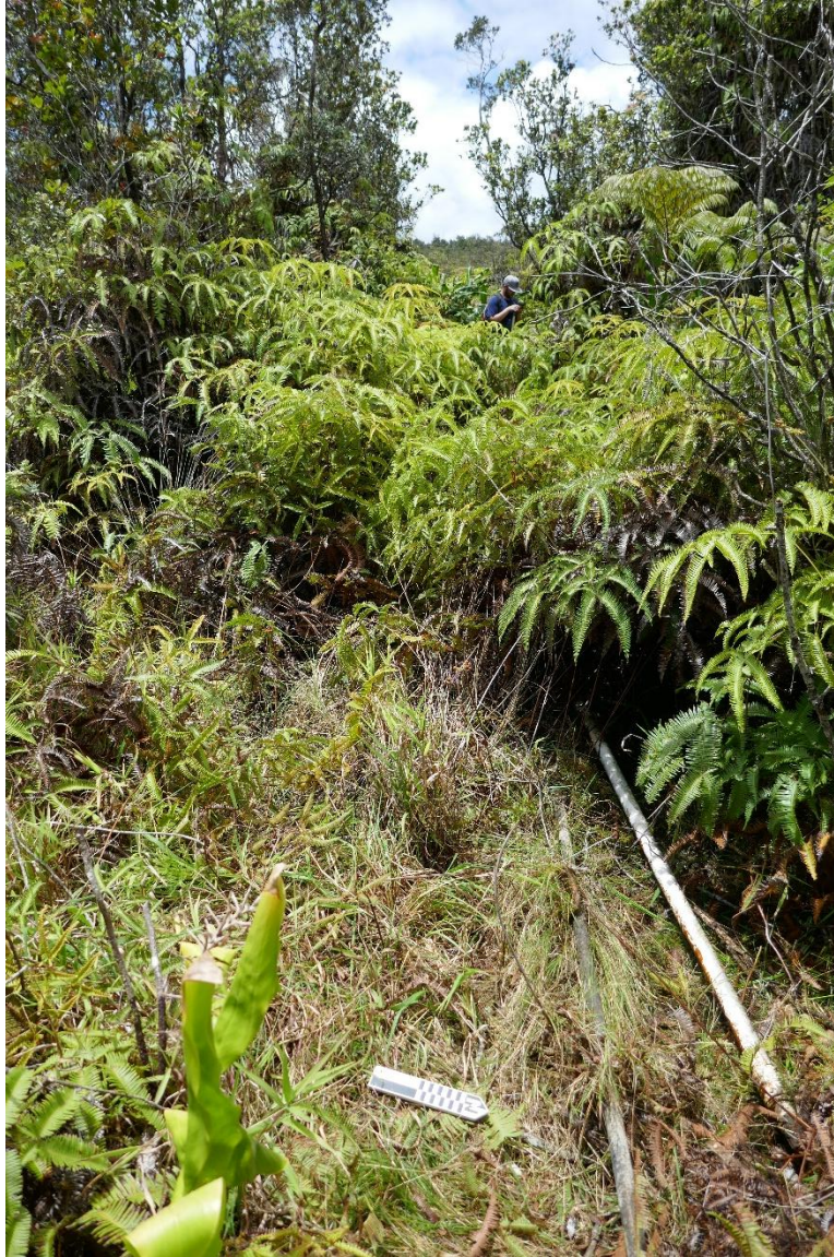
Photo 12 SIHP #50-xx-xx-xxxx2, water pipe lines laid along rail road bed at T8, view west.
