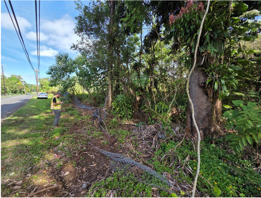
Photo 9: South end of the revised APE, on the east side of Kīlauea Avenue. Photo taken facing north. This image depicts part of the area added to the APE. Photo taken December 1, 2025.
