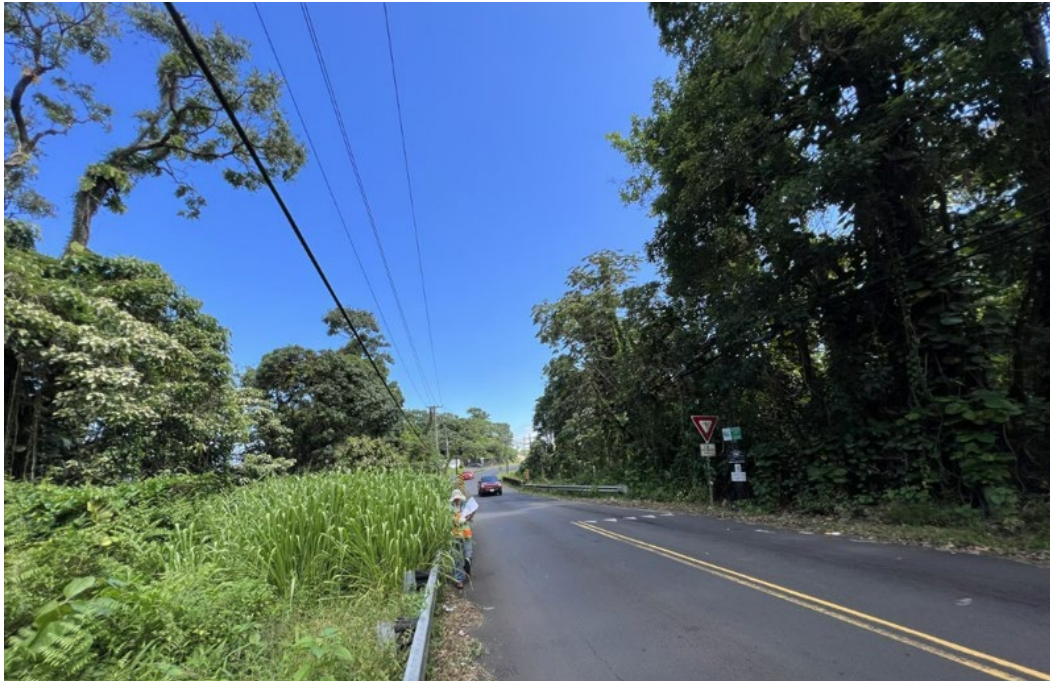
Photo 1: Photo of the southern approach to the one-lane Four Mile Creek Bridge. Photo taken from Kīlauea Avenue, facing north. Vegetation surrounding the bridge is weedy, introduced species, such as Guinea grass ( Megathyrsus maximus ) and African tulip tree ( Spathodea campanulata ). Photo taken June 11, 2024.
