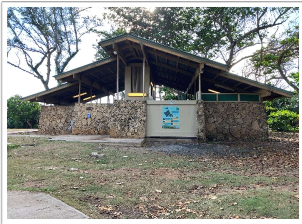
Figure 2-5 Photo of Comfort Station A
