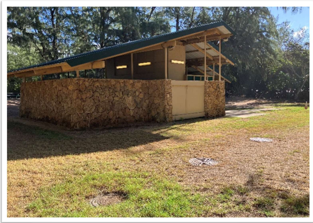
Figure 2-4 Photo of Comfort Station B
