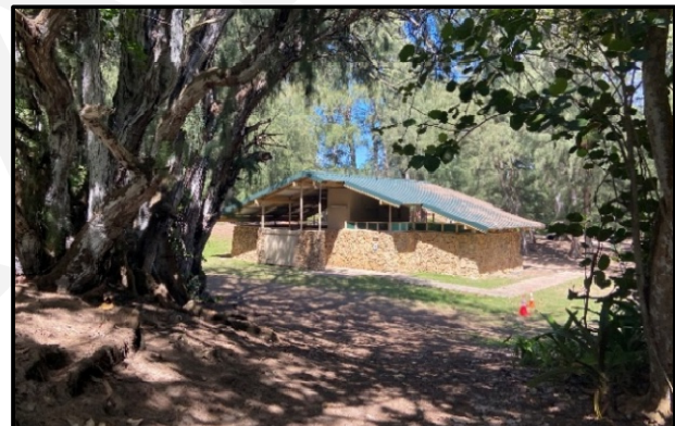
Photo 2 – Comfort Station B (Facing Southwest)
