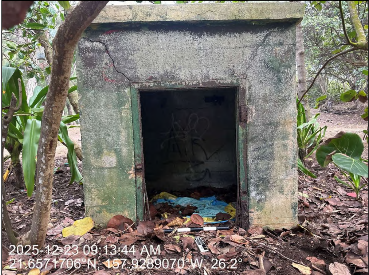
Figure 21. Detail of opening on south side of small concrete structure, possible military pillbox, near the southeastern boundary of the construction footprint; view north
