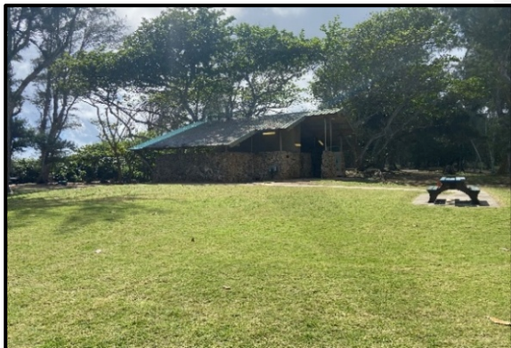
Photo 1 – Comfort Station A (Facing Southeast)
