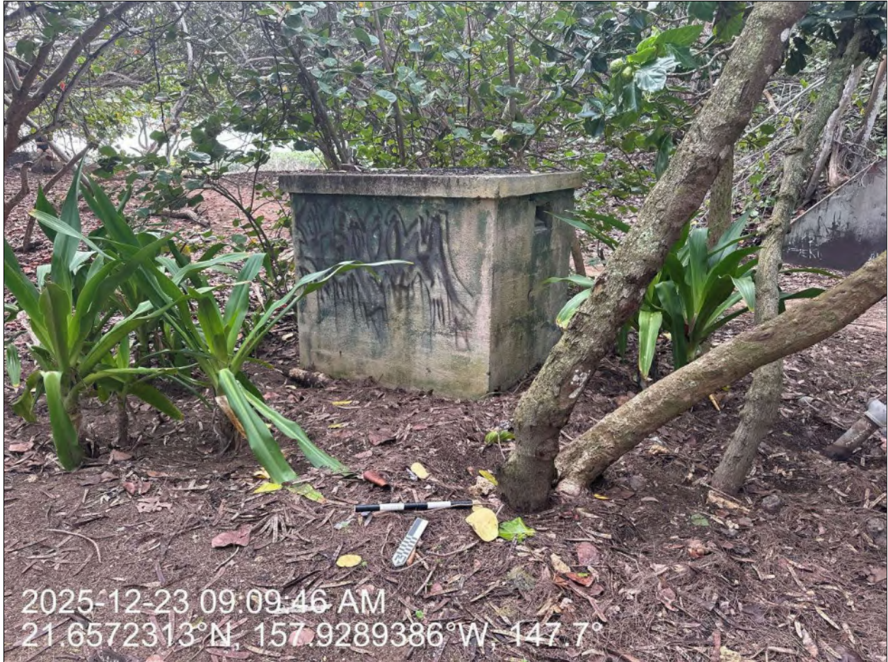
Figure 20. Another view of small concrete structure, possible military pillbox, near the southeastern boundary of the construction footprint; south-southeast
