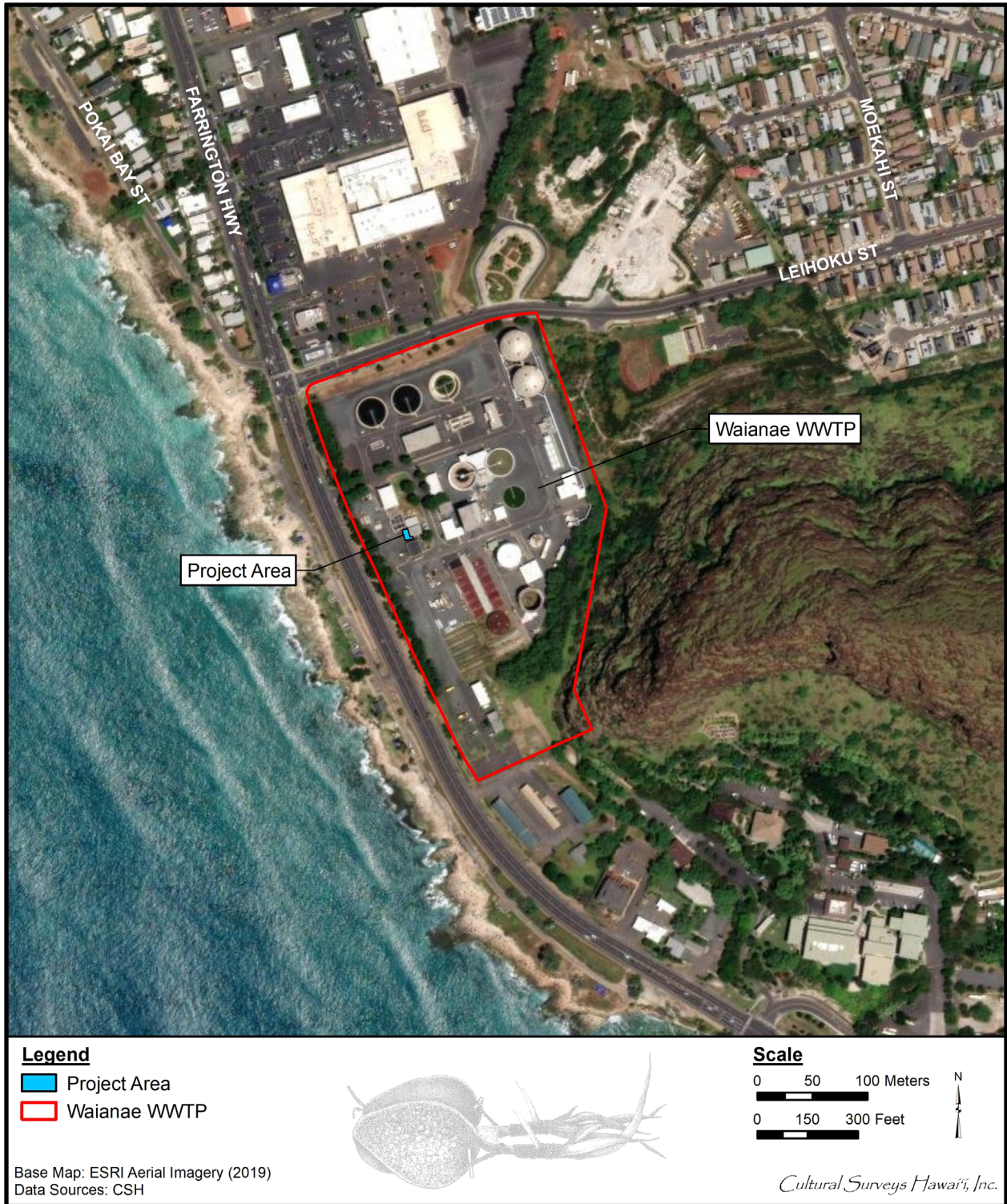
Figure 3. 2019 ESRI aerial photograph showing the Waianae WWTP and the location of the project area
