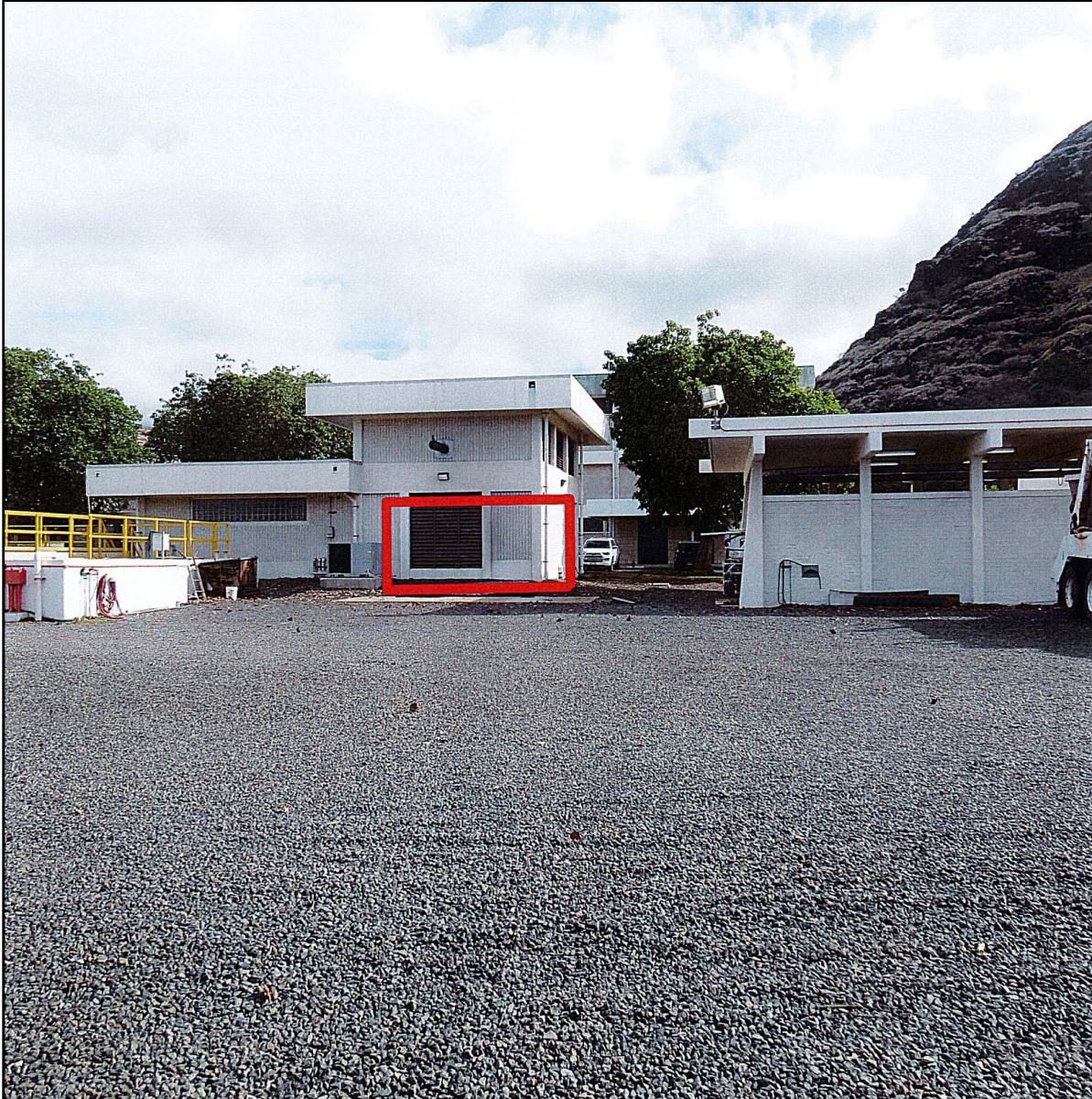
Figure 5. Photograph showing the location of the proposed new 6,000-gallon AST in the west central portion of the Waianae WWTP, at the location of an existing (to-be-removed) UST on the southwest side of a two-story Generator Building (at center) and just northwest of a Chlorination Building (at right), view to north (Okahara and Associates, Inc.; courtesy of client)
