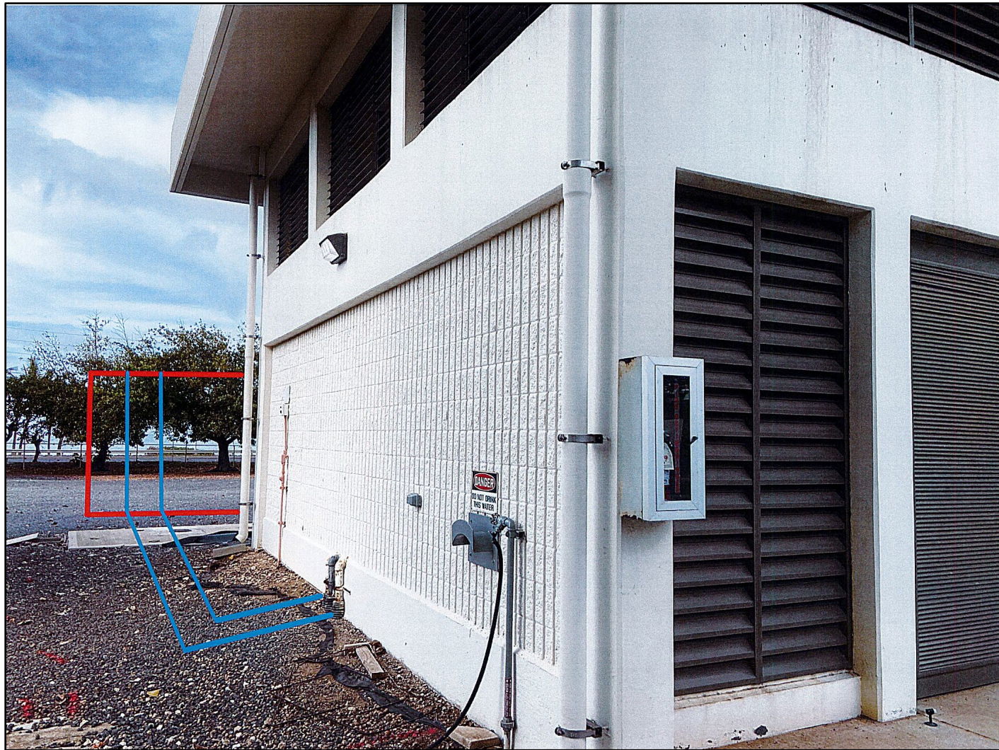
Figure 6. Photograph showing the location of the south end of the proposed new 6,000-gallon AST and new above ground fuel piping that will extend along a portion of the south side of the two-story Generator Building in the west central portion of the Waianae WWTP (Okahara and Associates, Inc.; courtesy of client)
