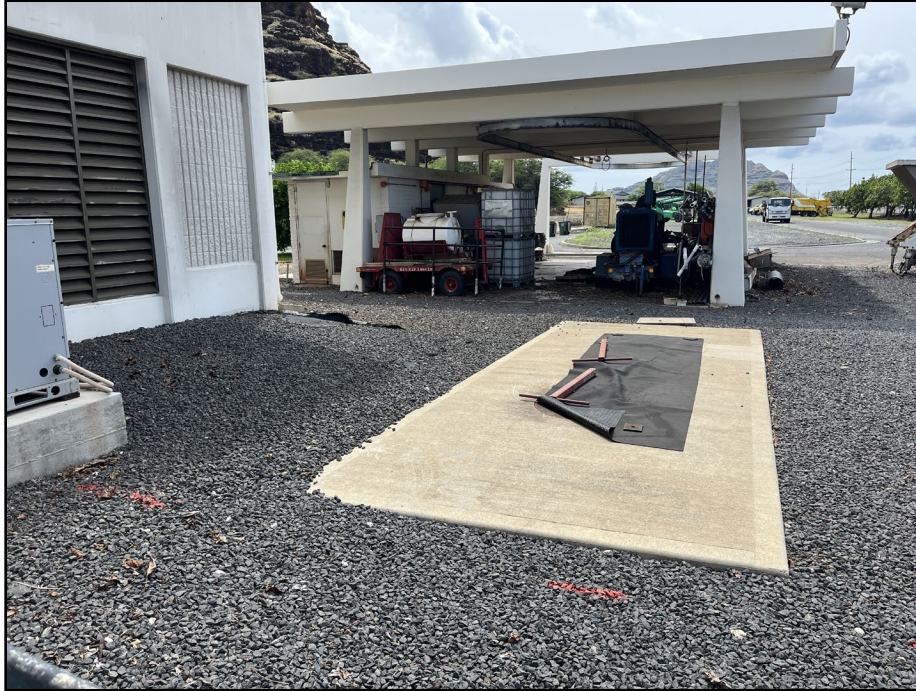
Figure 34. Photo C: View of the location of a new 6,000-gallon diesel AST at the location of a to-be-removed UST (under concrete slab), view to southeast
