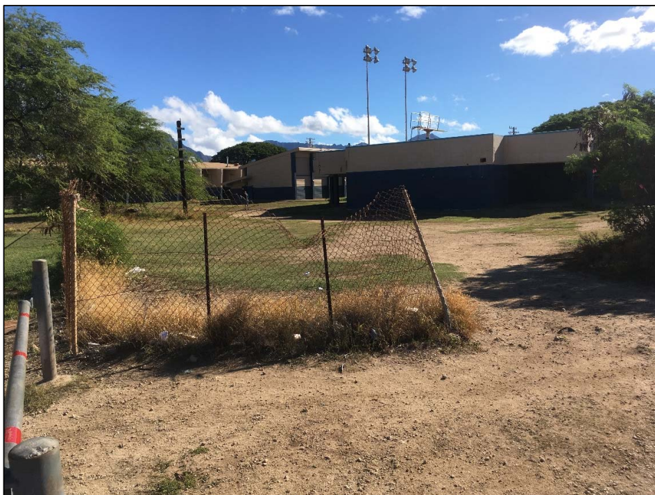
Figure 33. View of Access Road from beach to campus, above-ground pool in center, view to the north
