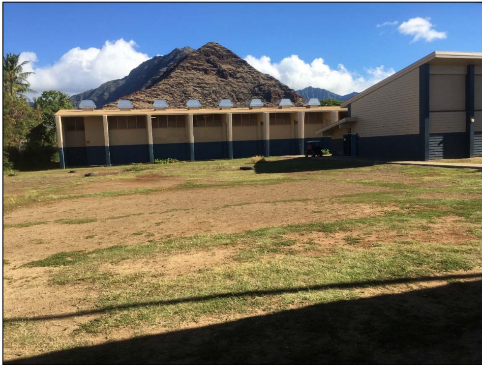
Figure 28. Gymnasium in back, Building T to right, view north
