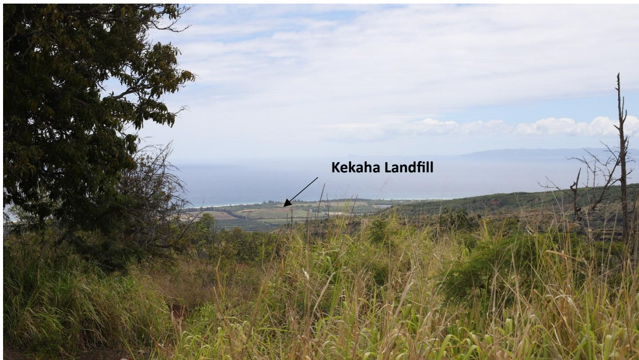
Photo 14. Upland view of Kekaha Landfill from Kokee Road.
