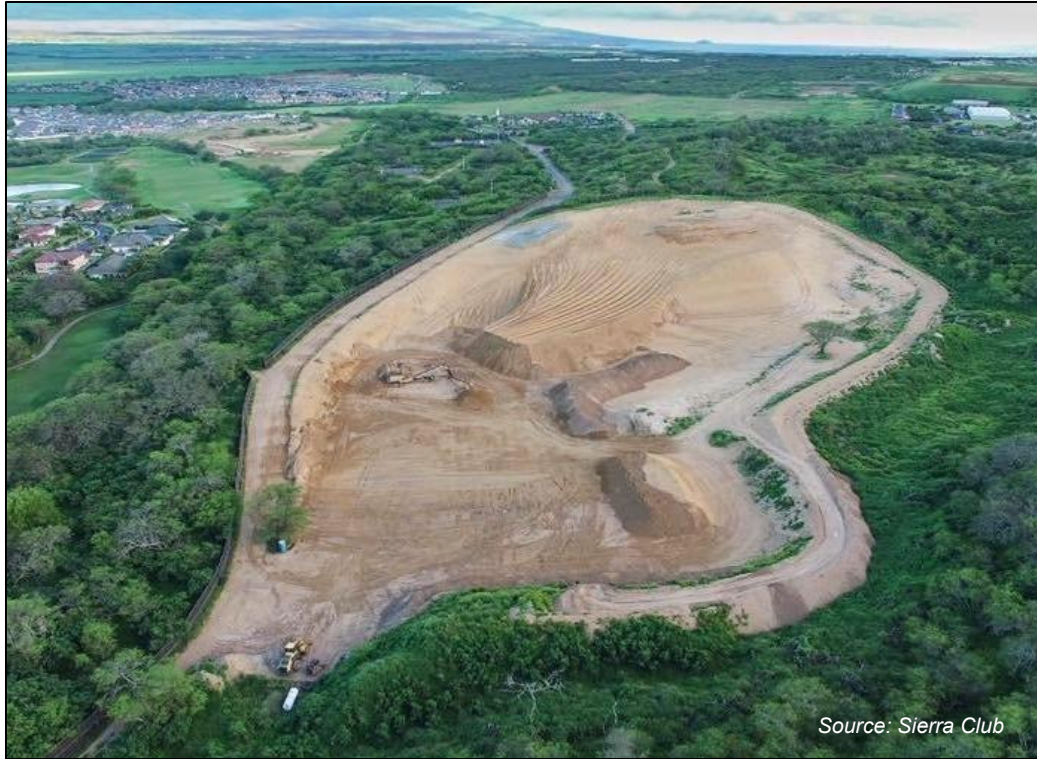
Figure 5-8 Excavation of inland dune sand at Maui Lani
