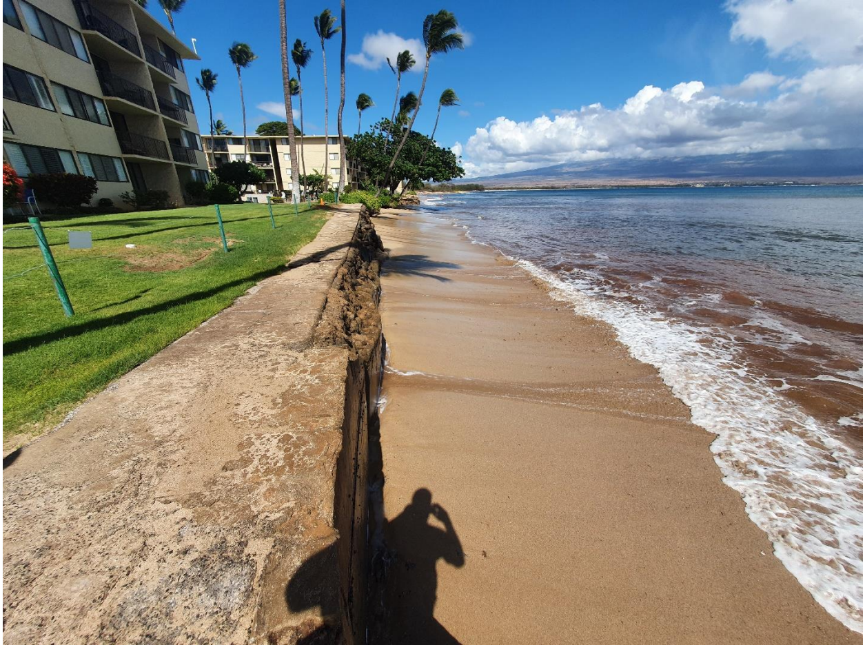
Photograph 13. Section 1 Seawall Looking East
