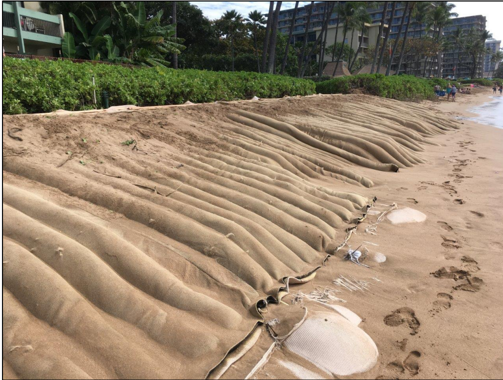
Figure 5-11 Geotextile sand filled mattress at Kaanapali, Maui (2018)
