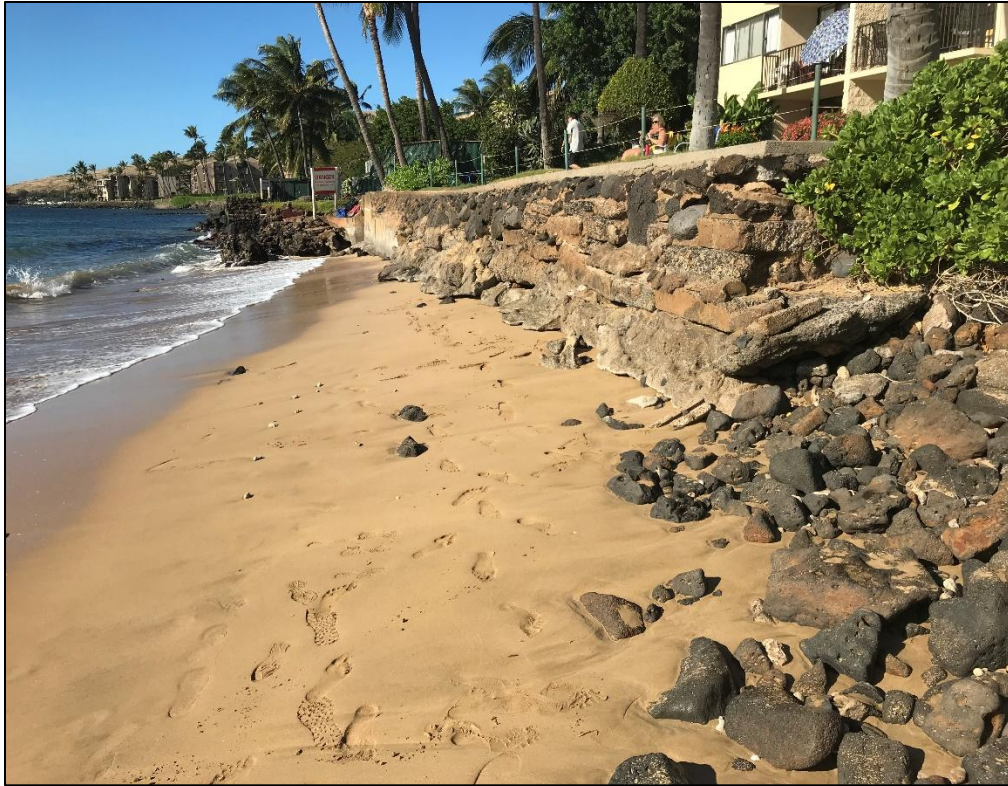
Figure 5-15 Existing CRM seawall at west end of KAN shoreline
