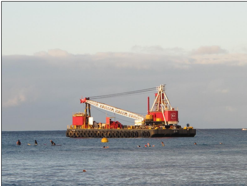
Figure 5-9 Offshore sand recovery at Waikiki Beach, Oahu (2012)
