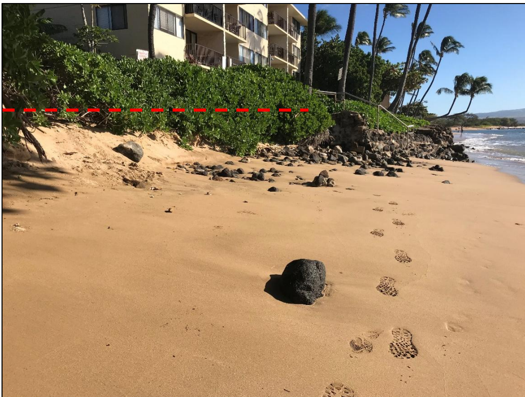
Figure 4-11 Approximate location of erosion scarp (dashed line)
