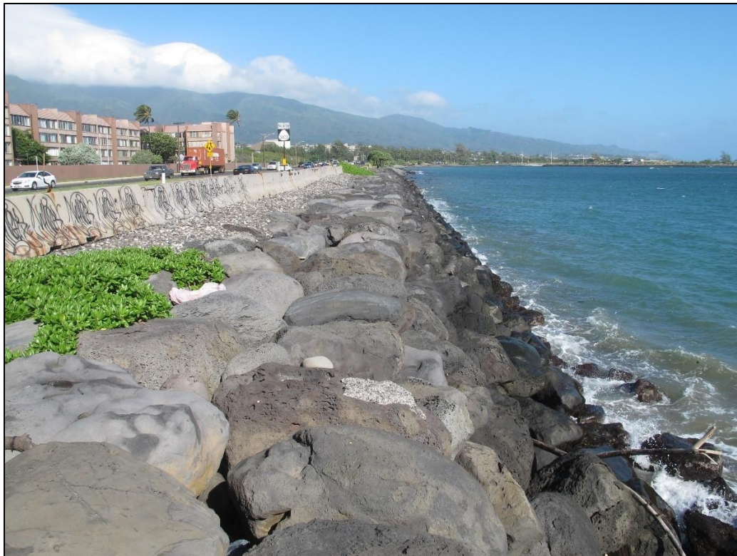
Figure 5-21 Rock rubblemound revetment at Kahului, Maui (2011)
