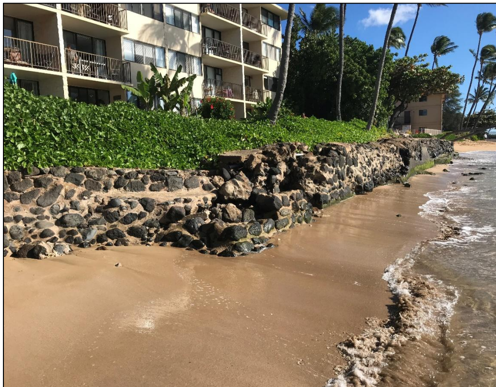
Figure 5-16 Existing CRM seawall at east end of KAN shoreline
