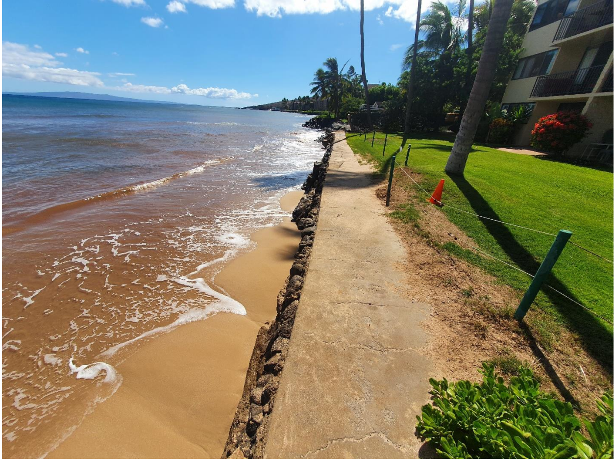
Photograph 14. Section 1 Seawall Looking West
