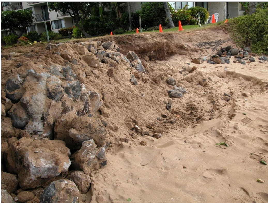
Figure 4-15 Removal of failed seawall section (2009)
