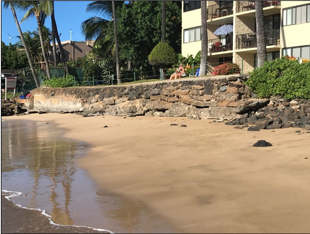
Figure 4-4 CRM seawall in Section 1 (west)
