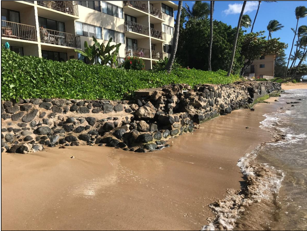
Figure 4-17 CRM seawall in Section 3 (east)
