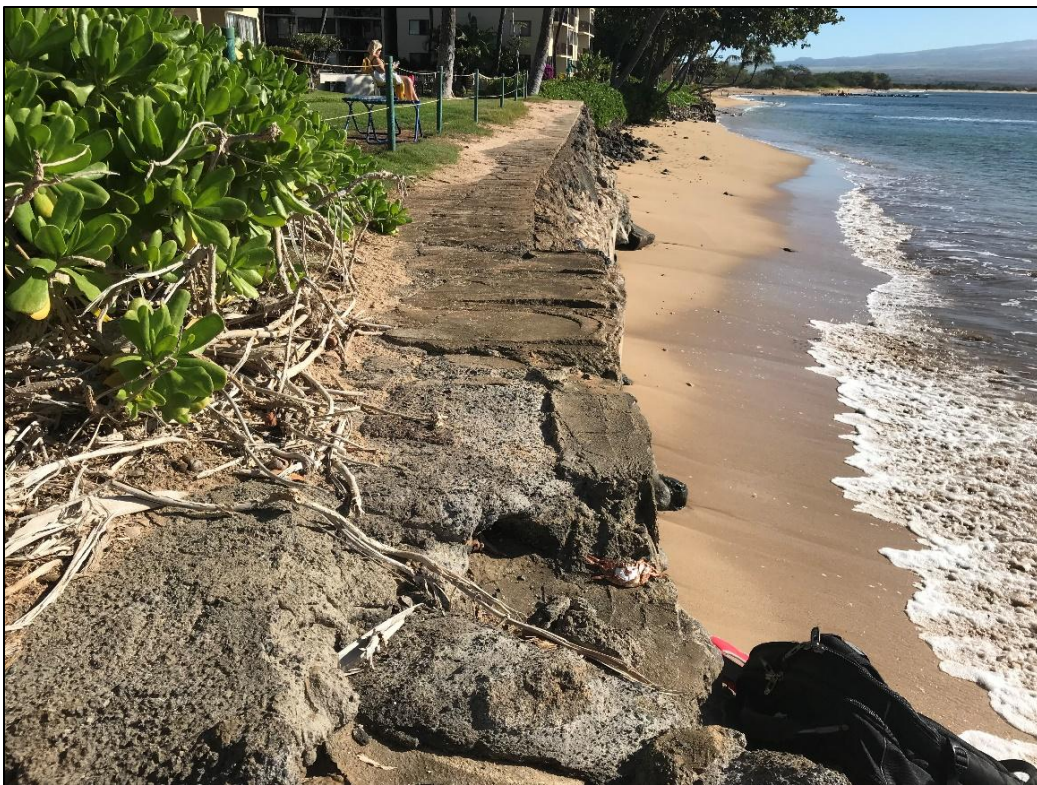
Figure 4-5 Concrete cap on top of seawall
