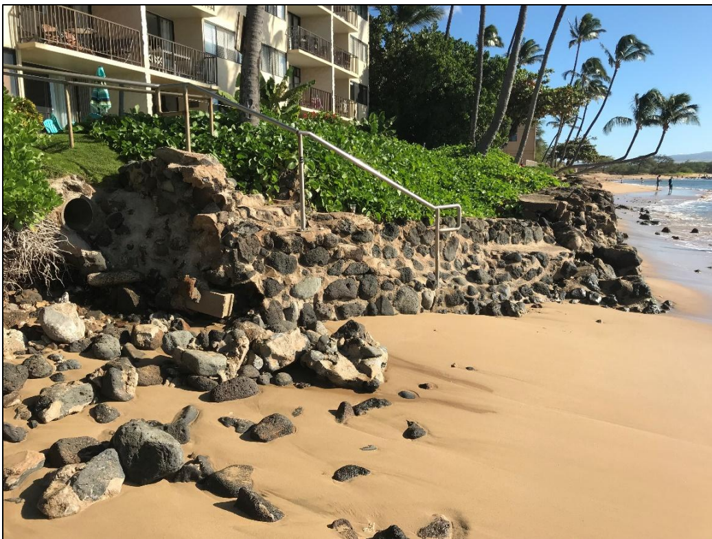
Figure 4-18 CRM stair at west end of seawall
