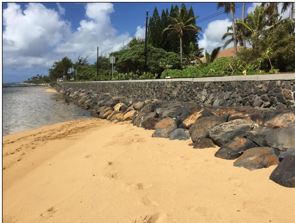
Figure 5-24 Hybrid seawall-revetment at Kapaa, Kauai (2012)
