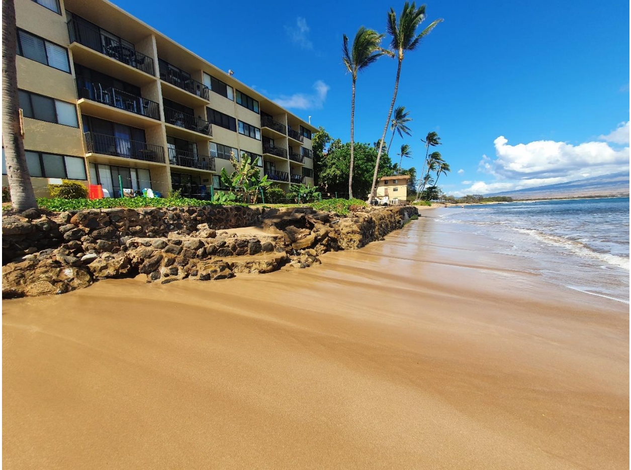
Photograph 18. Section 3 Seawall Looking East
