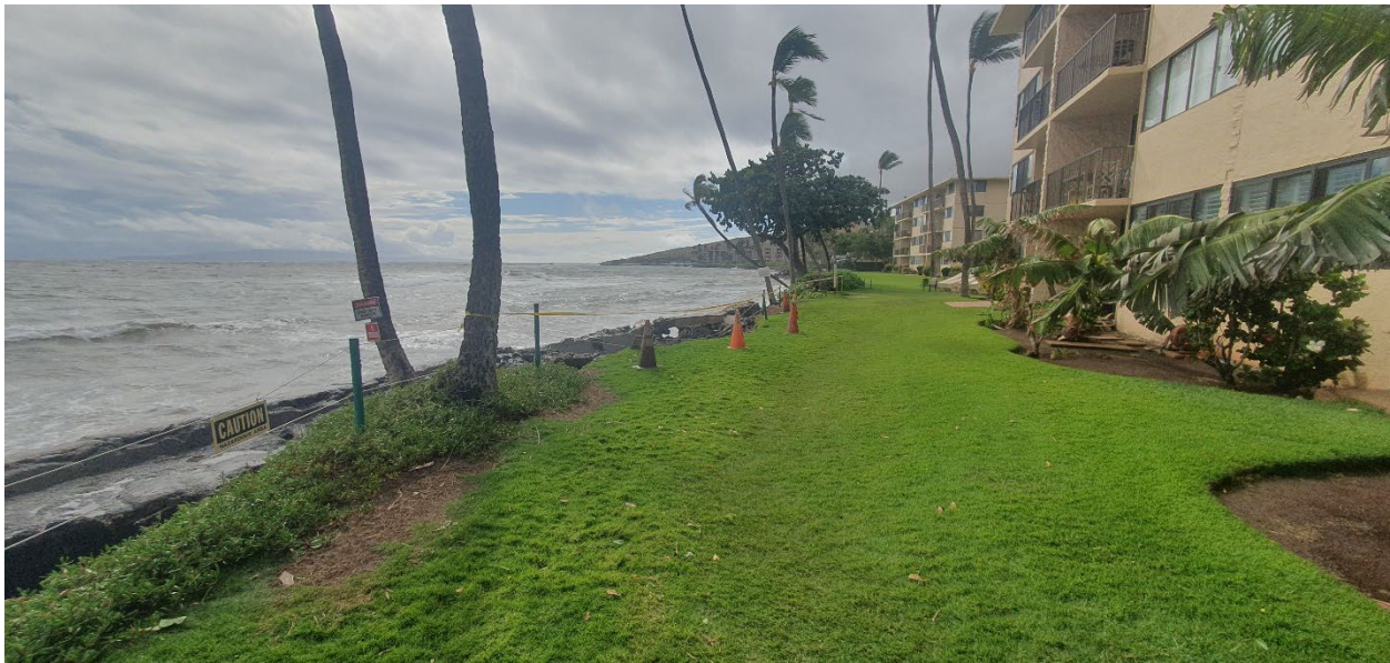
Figure 6: Rear Yard. Location of Geotextile Burrito Installation and Native Dune & Plant Restoration.
