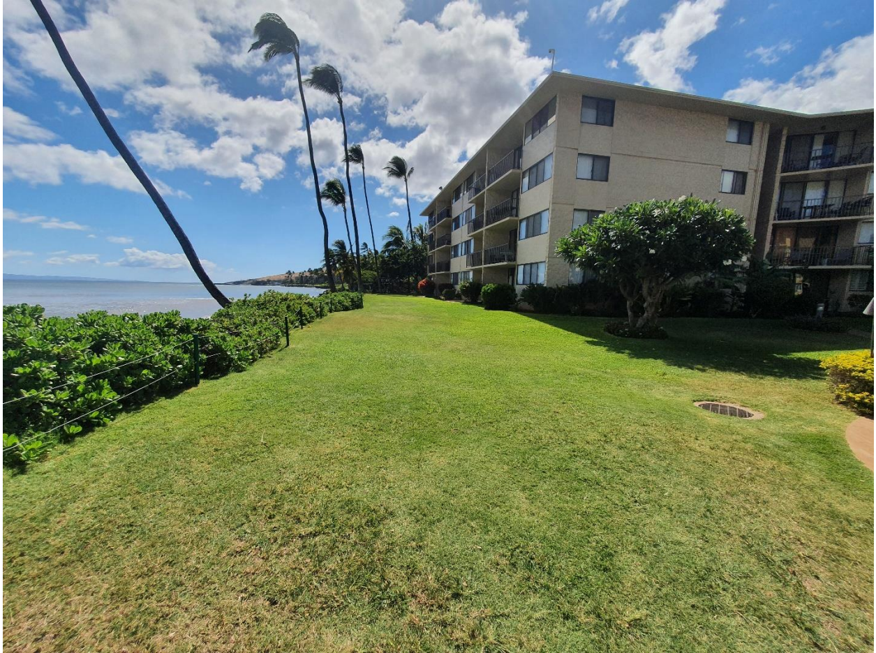
Photograph 11. Rear Yard Looking West - Pool to Right - – Location of Geotextile Burrito and Native Plant Dune.
