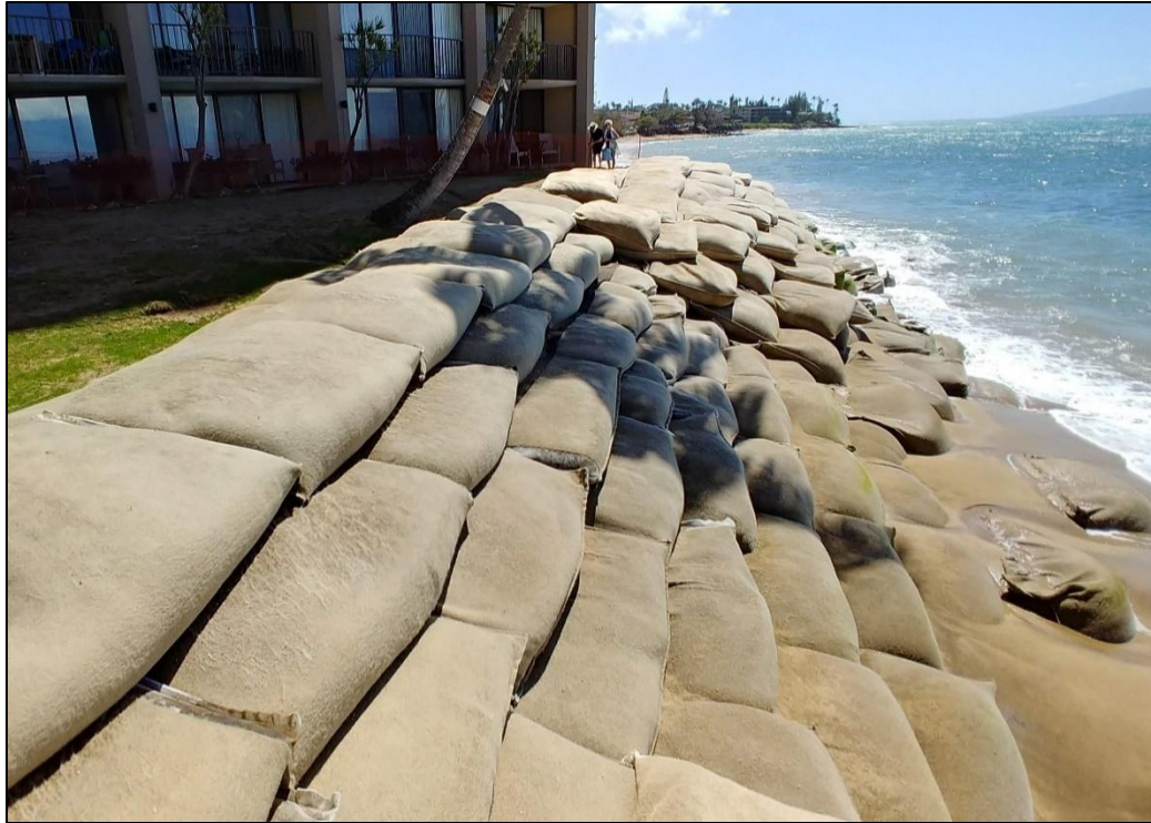
Figure 5-12 Geotextile sandbag revetment at Kahana, Maui (2018)
