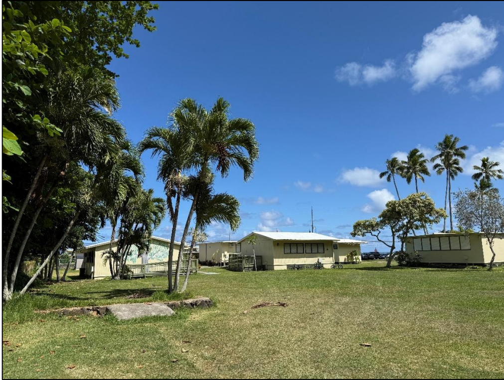
Figure 3. Lawn with scattered trees surrounding school buildings.
