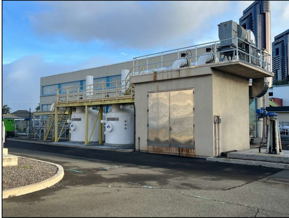
Figure 54. Photo O: View of the southwest side of the Ala Moana # 1 building, view to northeast
