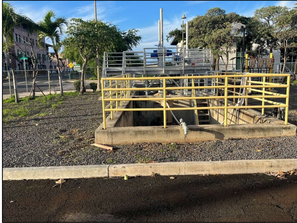
Figure 52. Photo M: View of infrastructure in the south corner of the Ala Moana No. 1 WPS, view to southwest
