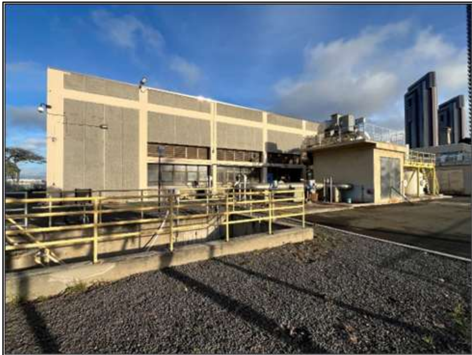
Figure 51. Photo L: View of the southeast side of the (1983) Ala Moana # 2 building, view to north
