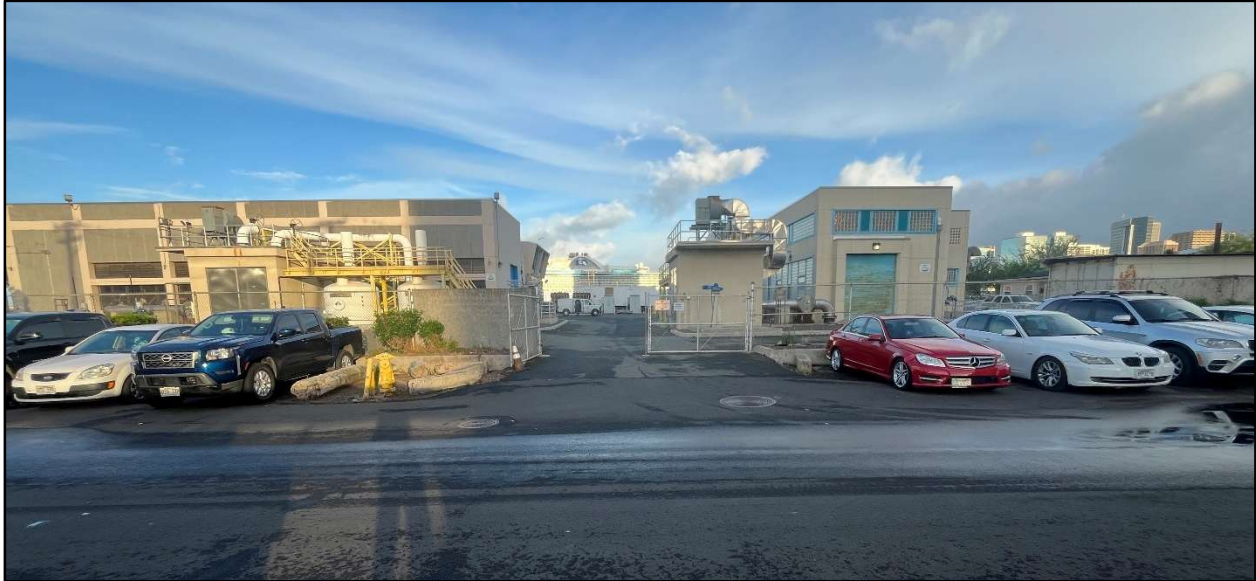
Figure 40. Photo A: View of entrance gate to the Ala Moana No. 1 WPS Improvements project area at 210 Keawe Street from across Keawe Street, view to northwest
