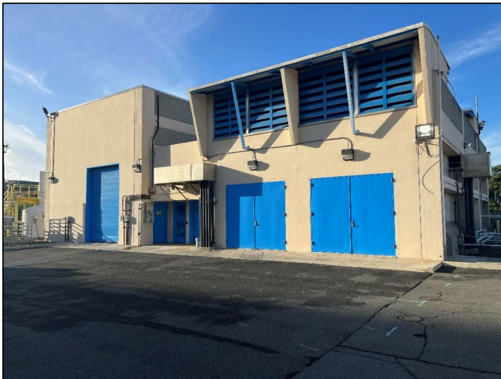
Figure 57. Photo R: View of the northeast side of the Ala Moana # 2 building, view to southwest
