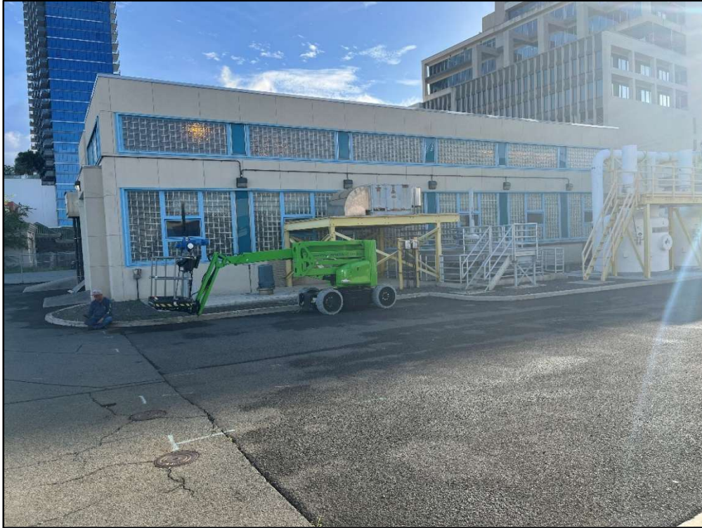
Figure 56. Photo Q: View of the long southwest side of the Ala Moana # 1 building, view to east
