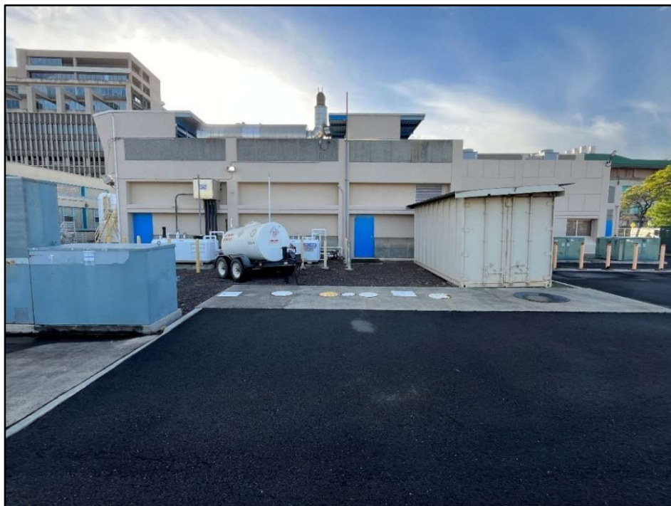
Figure 47. Photo H: View of the northwest side of the (1983) Ala Moana # 2 building (this is the portion of the facility understood as the focus of the Improvements Project), view to southeast
