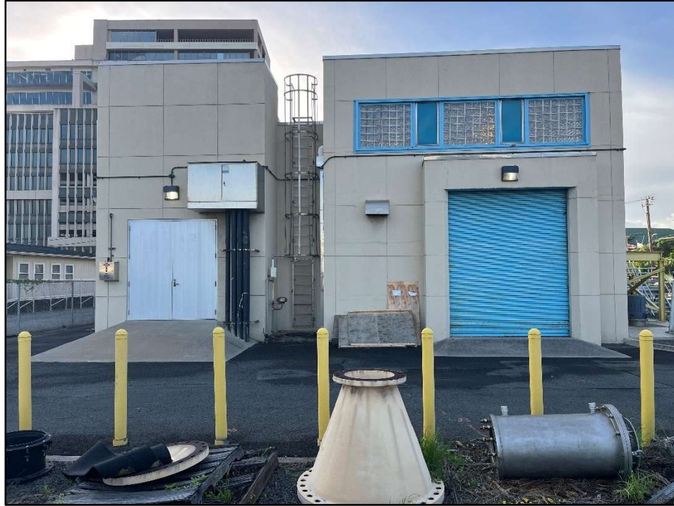
Figure 46. Photo G: View of the northwest end of the (1954) Ala Moana # 1 building, view to southeast
