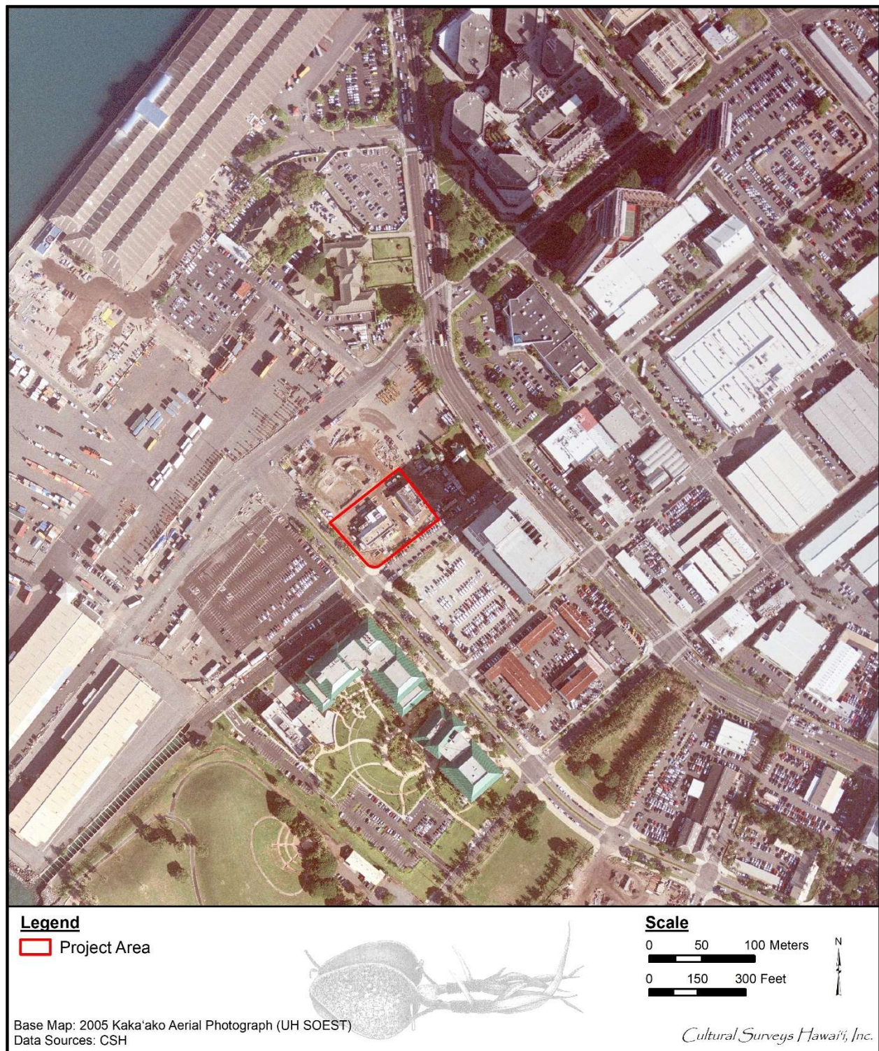
Figure 36. Portion of 2005 Kakaako aerial photograph (UH SOEST) showing the location of the Ala Moana No. 1 WPS Improvements project area much as it is today
