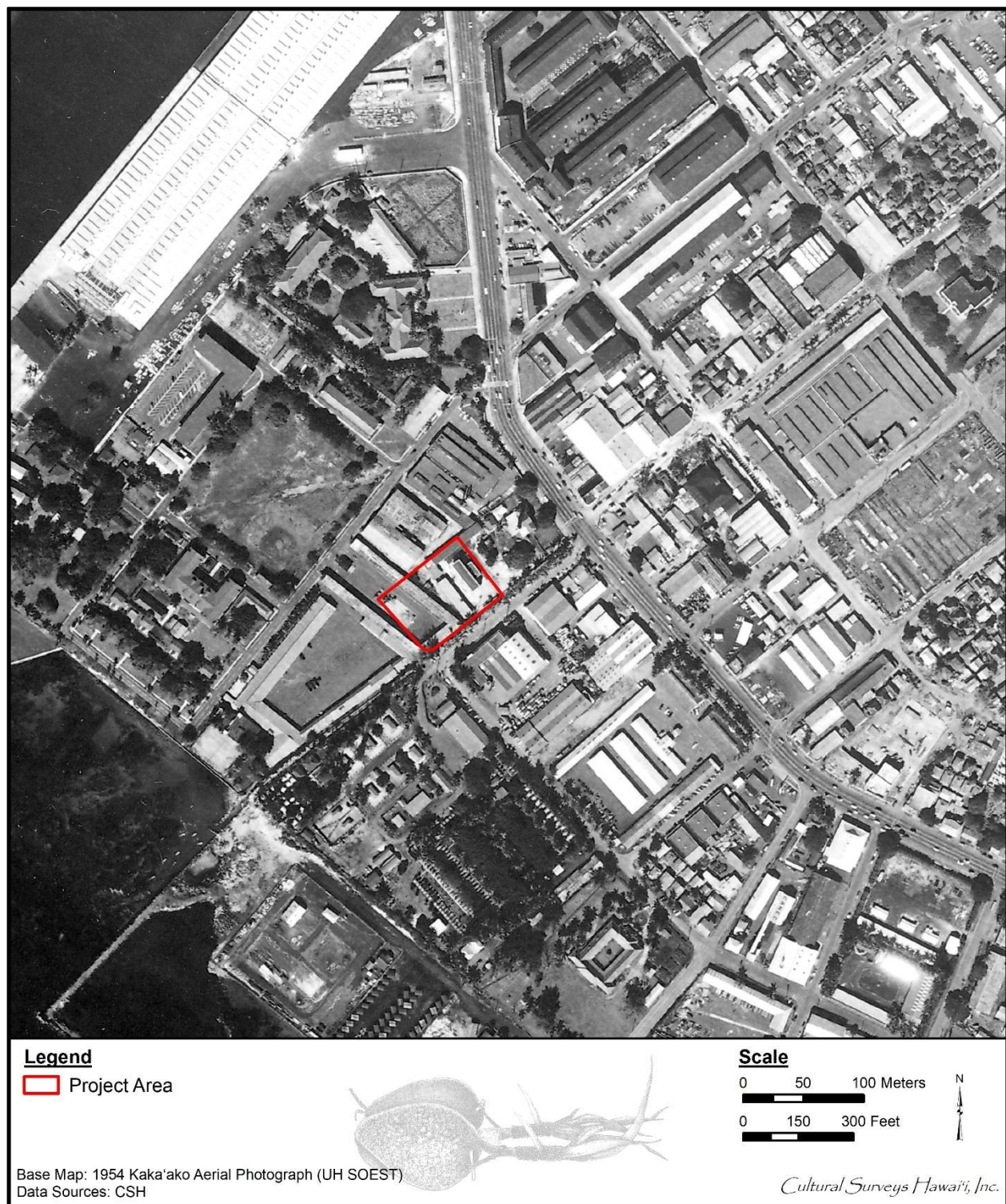
Figure 30. 1954 Kakaako aerial photograph (UH SOEST) showing the location of the Ala Moana No. 1 WPS Improvements project area which appears to show the brand new (1954) Ala Moana #1 building (rectangular northwest/southeast-oriented building in the northeast/central portion of the project area, still extant today)
