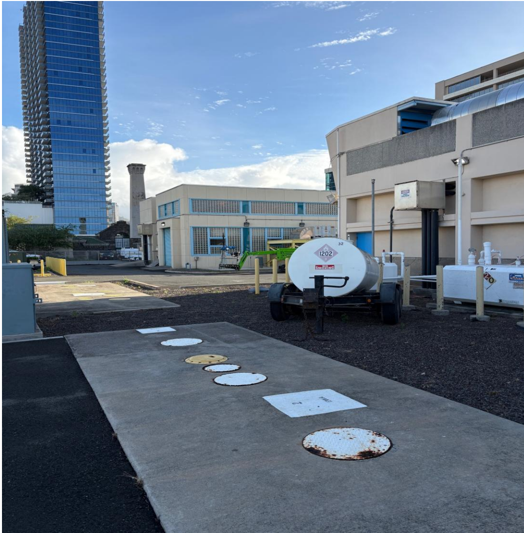
View of the proposed location for the AST behind Ala Moana No.2 WWPS (Ala Moana No.1 WWPS is in the background)
