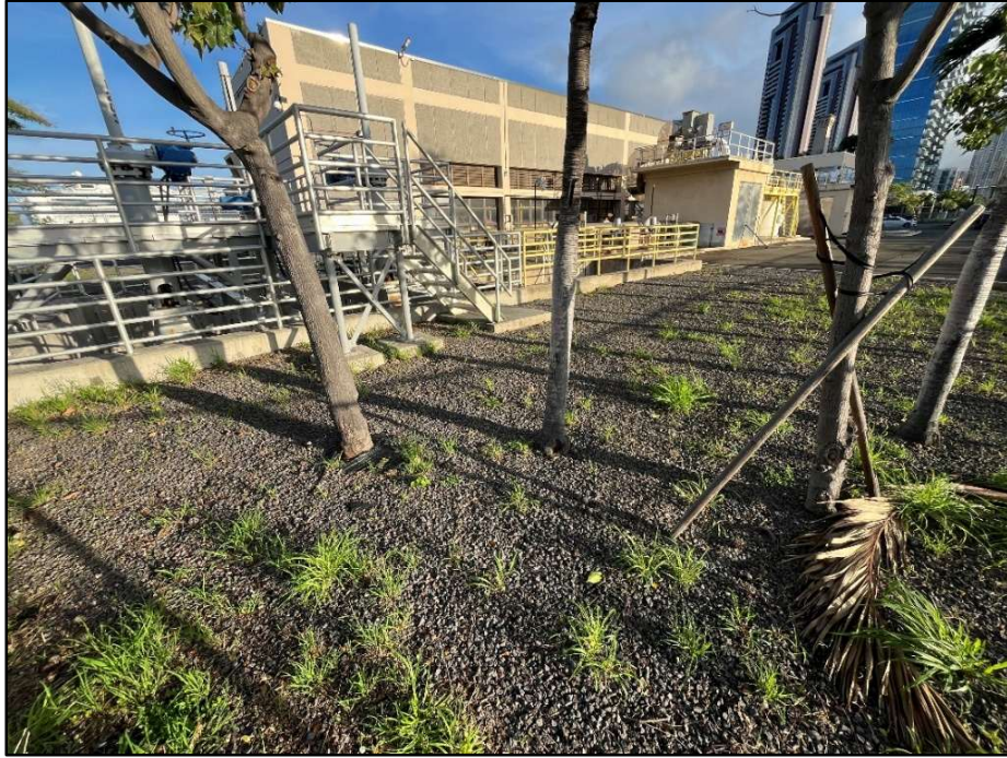
Figure 50. Photo K: General view from the south corner of the Ala Moana No. 1 WPS Improvements project area, view to northeast
