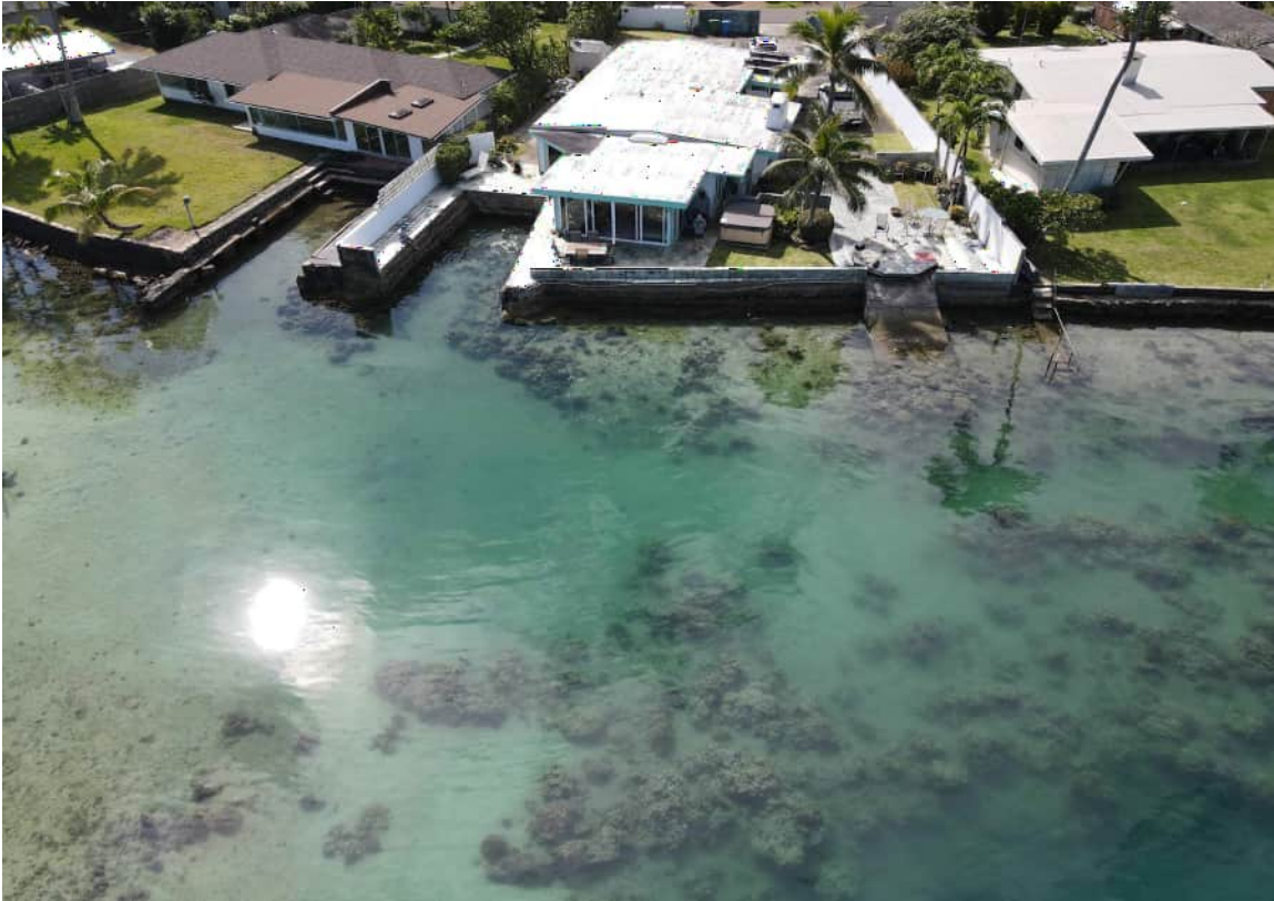
Figure 1-4. Aerial View of Marine Environment at the Project Site.
