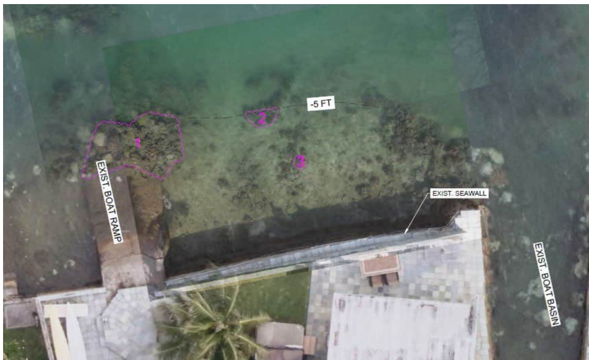
Figure 1-2. Aerial View of Project Area
