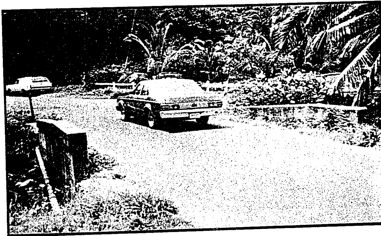
Plate 17 The Haena "Bridge" number 1 looking west. Note the settlement of the west abutment.
