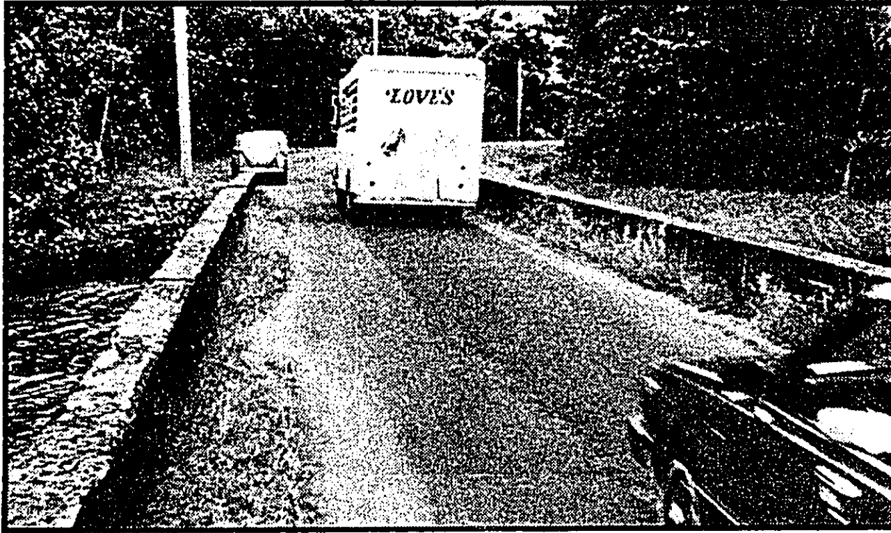
Plate 13 Cars waiting to cross the Waipa Bridge.
