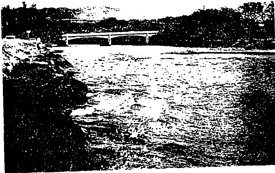
PLATE 7 (above): UngROUTED riprap revetment below highway bridge (background). View facing NE.
