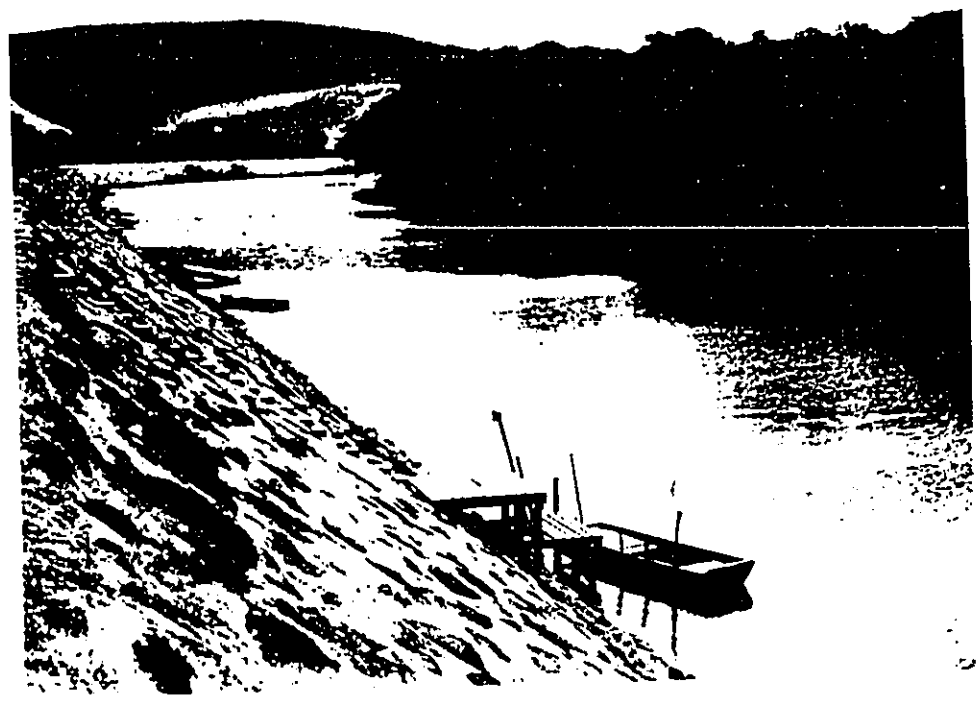
PLATE 4 (below): Middle reach of the existing levee. View facing NNE.
