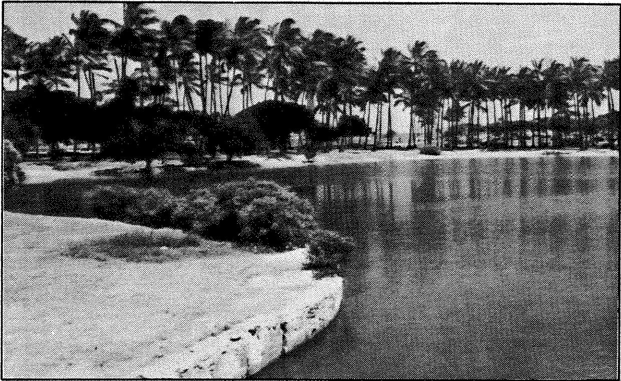
Plate 4 View across the first lagoon from the end of the canal looking toward the site of the new outlet channel.
