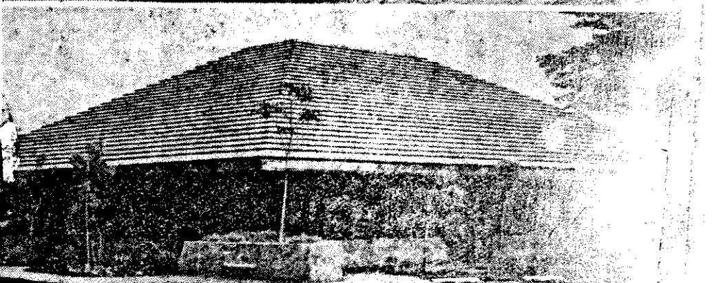
When First Hawaiian Bank outgrew its old Haleiwa quarters (top), it copied the building in an enlarged version (below).
