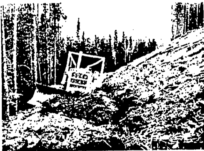
Figure 4-38. Extensive grading is required to create a level working area in steep terrain as shown in this example of a natural gas pipeline construction project.
