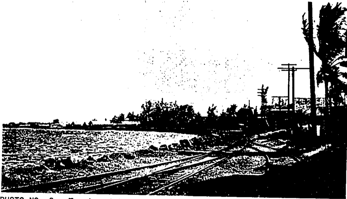
PHOTO NO. 2. Tracks with riprap stone revetment wall, Hilo Bay.
