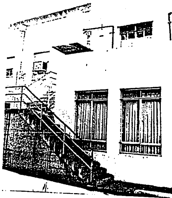
FIGURE 14 MTL OFFICE BUILDING—NORTH SIDE, 1987
