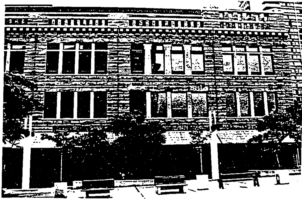
PHOTO F MODEL/PROGRESS BLOCK
