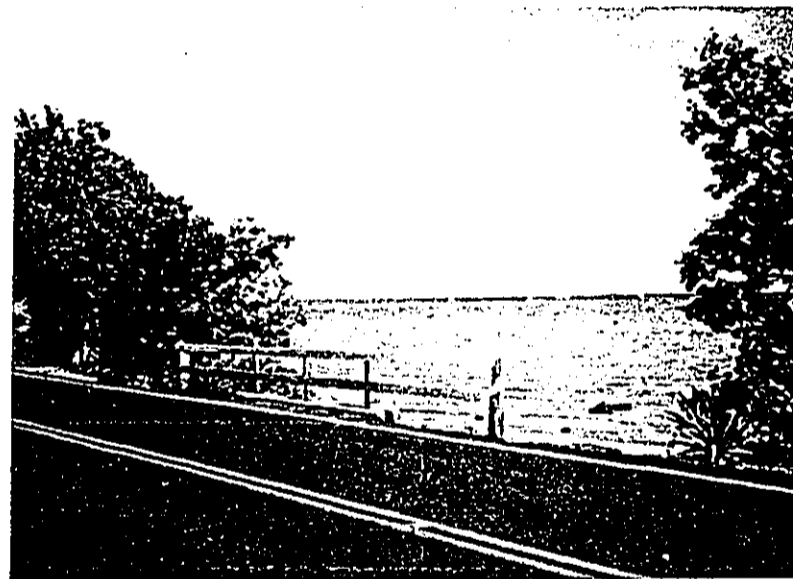
⑤ Opening in Vegetation at Drainage Outlet
