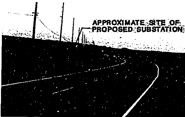
TYPICAL VIEW SOUTH ALONG QUEEN KAAHUMANU HIGHWAY, WITH POWER LINES MAUKA OF HIGHWAY, SHOWING APPROXIMATE SITE OF OOMA 2 HELCO/HTCO SUBSTATION
