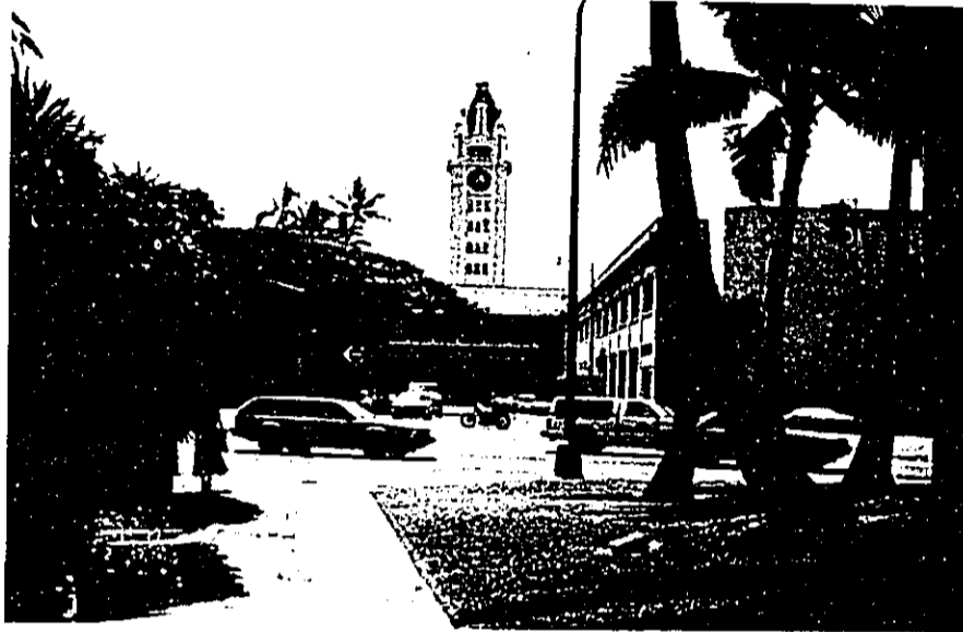
Aloha Tower's base is currently blocked from view down Fort Street. The project proposes to open this view channel through the base of Aloha Tower to the harbor beyond. The Aloha Tower Hotel will be located at right; the refurbished Irwin Park at left.
