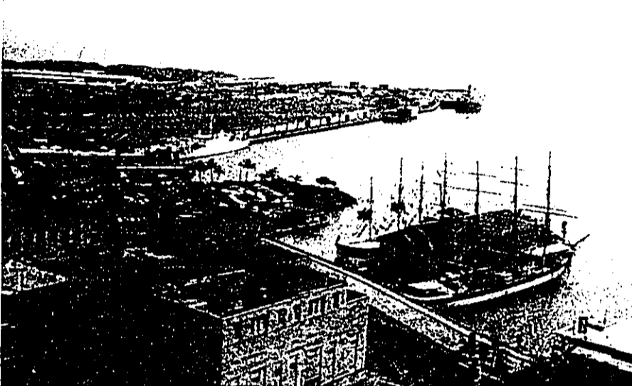
View of Piers 5, 6, and 7. Piers 5 and 6 will be extended to accommodate new Maritime Building and Passenger Terminal. Pier 7 will remain as is, with the addition of the Duke Kahanamoku Water Sports Center at the mauka end. The existing ramp will be demolished.
