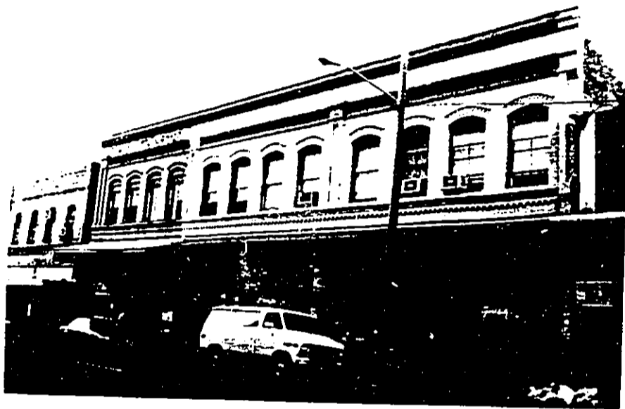
Photo 15. Remainder of Y. Anin Building
