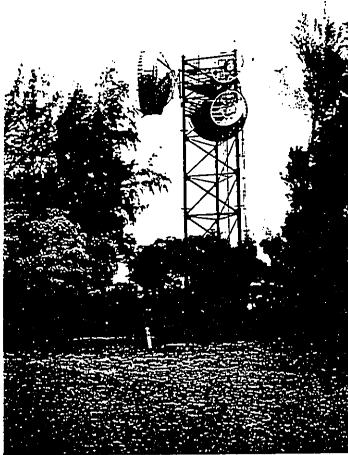
Existing 70-foot antenna tower with microwave repeater station at lower left of tower.
