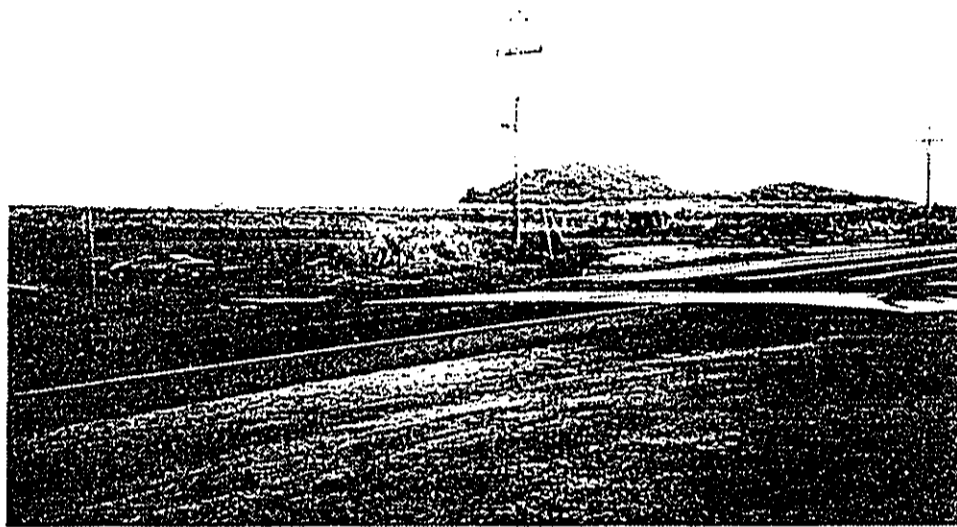
Photo 1. View of the site. Looking North from across Kapule Highway.
