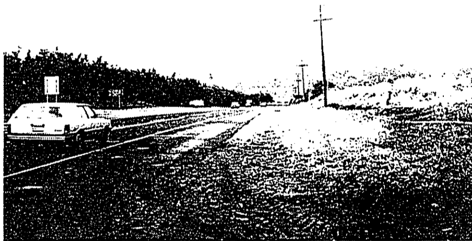
Photo 2. View of the site and Kapule Highway. Looking southwest.
