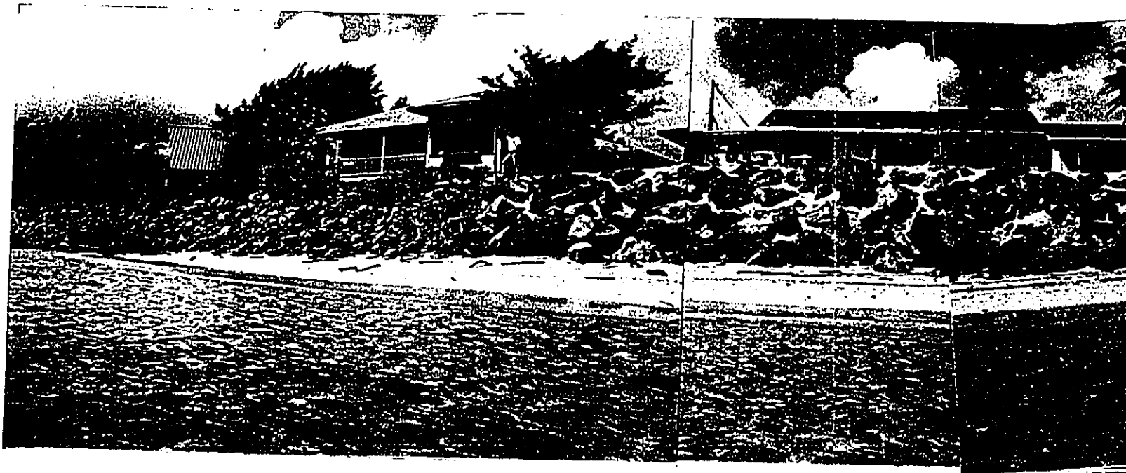
This panoramic view shows the revetment in front of TMK 5-5-2:85 which was constructed in August 1991. At 5-2:32; just visible to the right is the end of the revetment in front of TMK 5-5-2:30. Sand has accumulated at the top (horizontal) slope.
