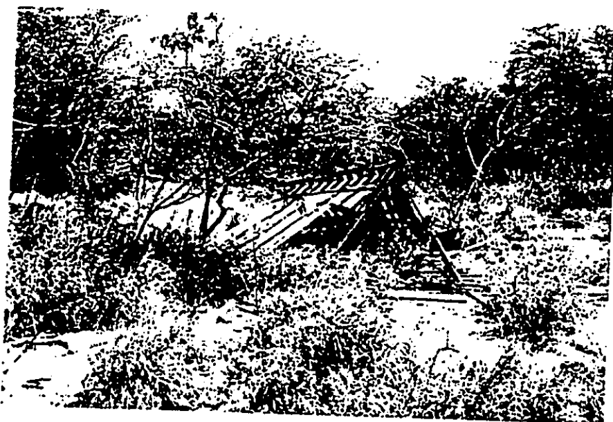
Fig. 13. SITE 50-Ma-C1-15, HISTORICAL BUILDING. View to Southwest. BM Neg. No. Ma(a)340-25.
