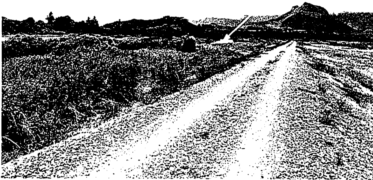
PHOTO 5: SOUTHERN VIEW FROM LEVEE STATION 65+00.
