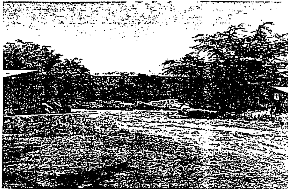
Figure 8 Mauka Portion of Cable Corridor Showing Graded Area. Facing Mahai
