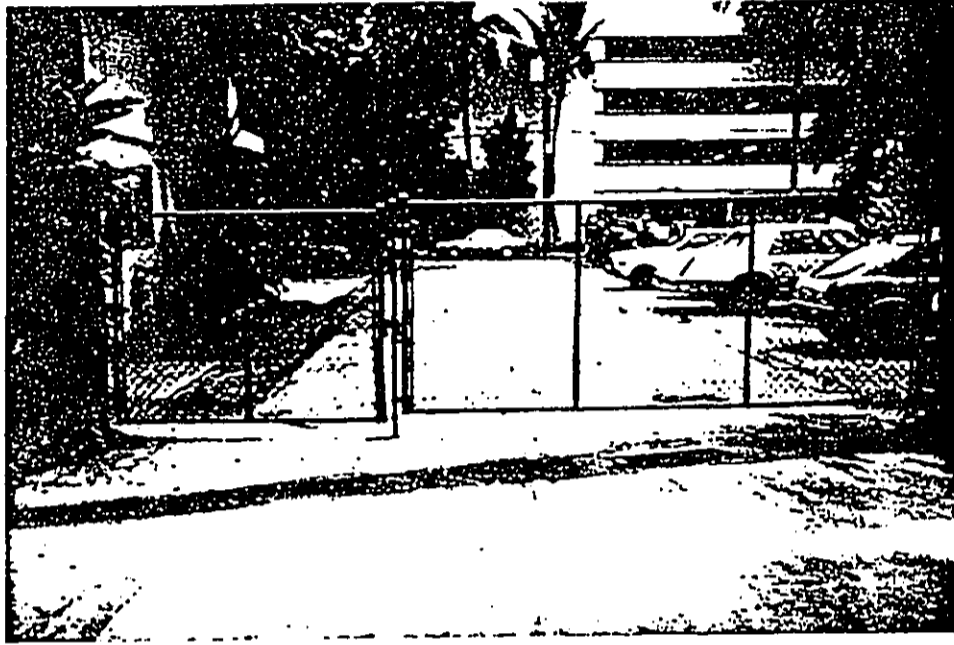
Gated entry way to the ground floor parking stalls (Looking towards Kaioo Drive)
