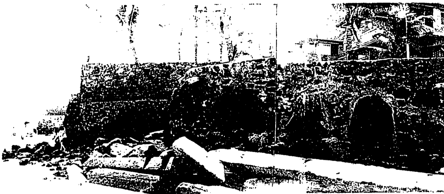
Figure 6 : Close view of beach park's seawall fronted by boulders, spall material and concrete piles. (2/93)
