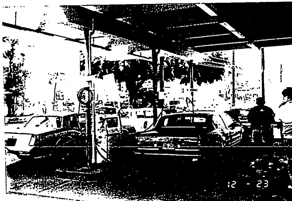
Two dispenser pumps at Police Motorpool Facility.
