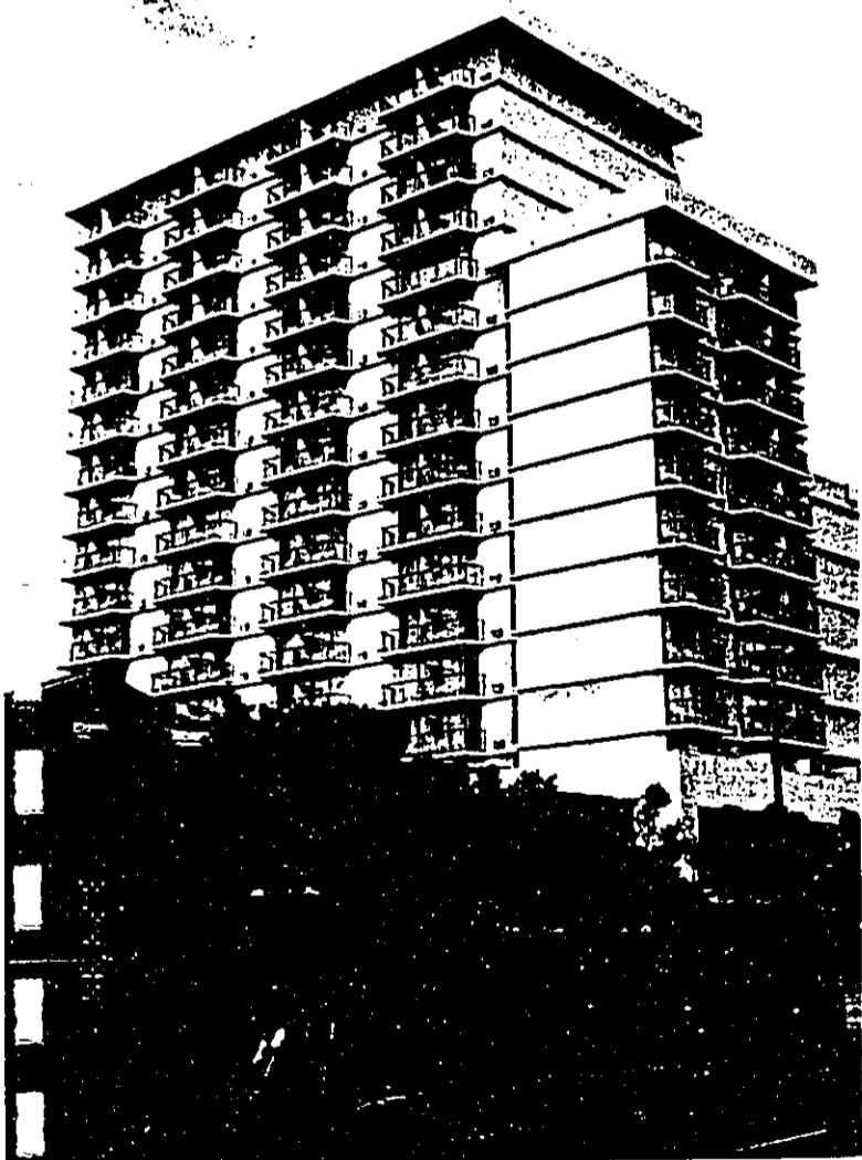
DIAMOND HEAD ELEVATION LOOKING FROM KALAKAUA AVE (SOUTHEAST)
