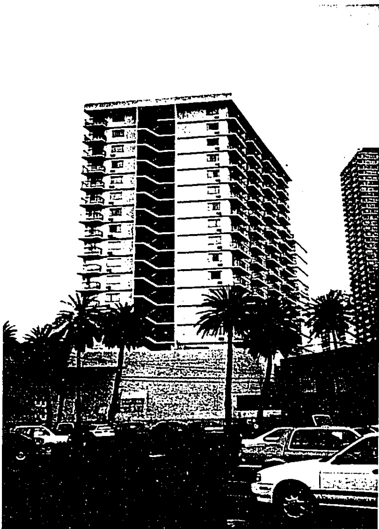
MAKAI ELEVATION LOOKING FROM FT. DERUSSY PARKING LOT (SOUTHWEST)
