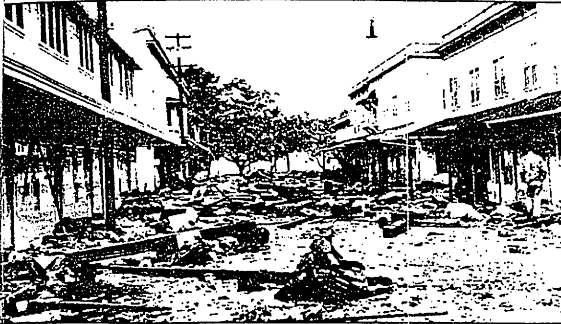
Debris litters the streets of Hilo after the 1946 tsunami, Hawaii's worst tsunami to date.
