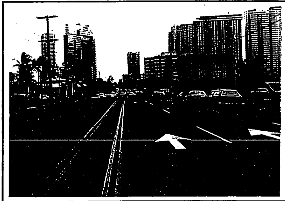
Kalakaua Avenue approach to Kapiolani Boulevard facing southeast.
